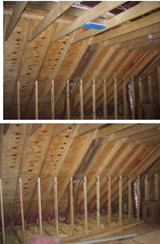
Figure 5. Supply register for attic space (top photo) and supply duct descending to ceiling register for second floor (bottom photo)
