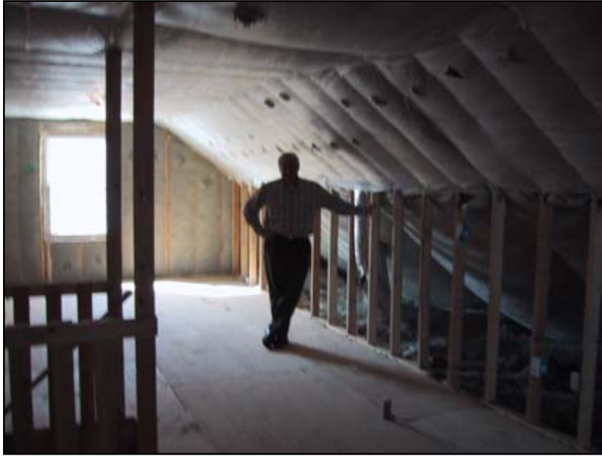
Figure 6. Alden Hathaway and blown-in cellulose insulation in attic
