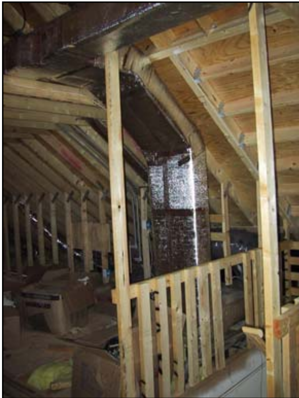
Figure 4. Duck supply trunk entering attic and continuing to trunk above the framing for the finished space
