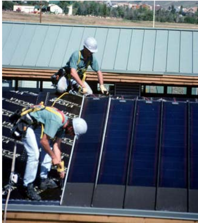
Figure 5-9 Installation of the roof-integrated PV panels
