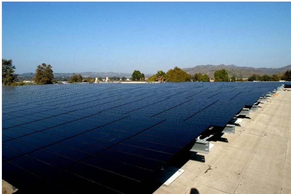
Figure 30. SSI's new 245 kW CIS thin film array.
