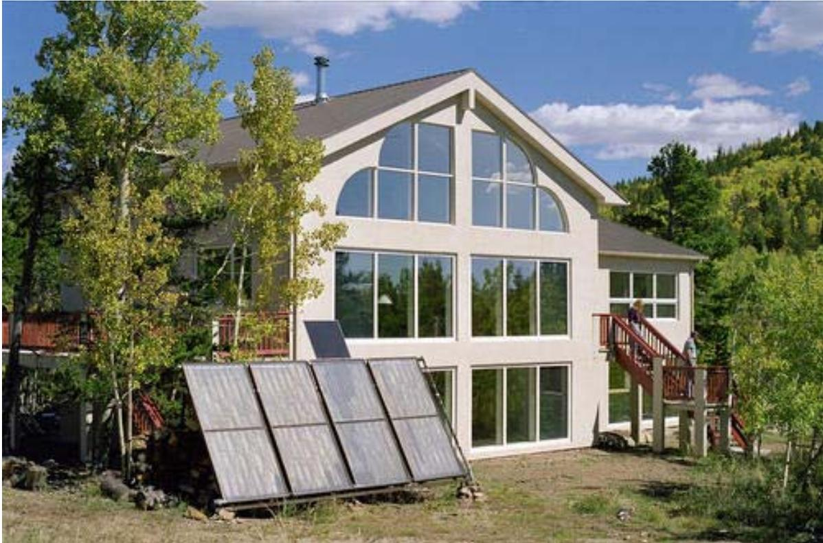
**The Van Geet home in the Rocky Mountains west of Denver, Colorado. This view from the southwest shows the south-facing glazing for passive solar heating and the solar hot-water collectors in the foreground. The 1,000-watt photovoltaic array east of the house is not shown in this view (NREL/PIX 08226).**
