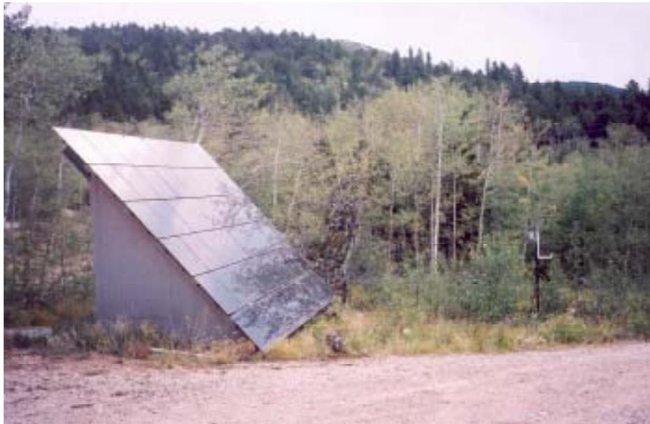
**Figure 6.4. PV array (shown as roof of shed) and weather station (located on right of photo)**
