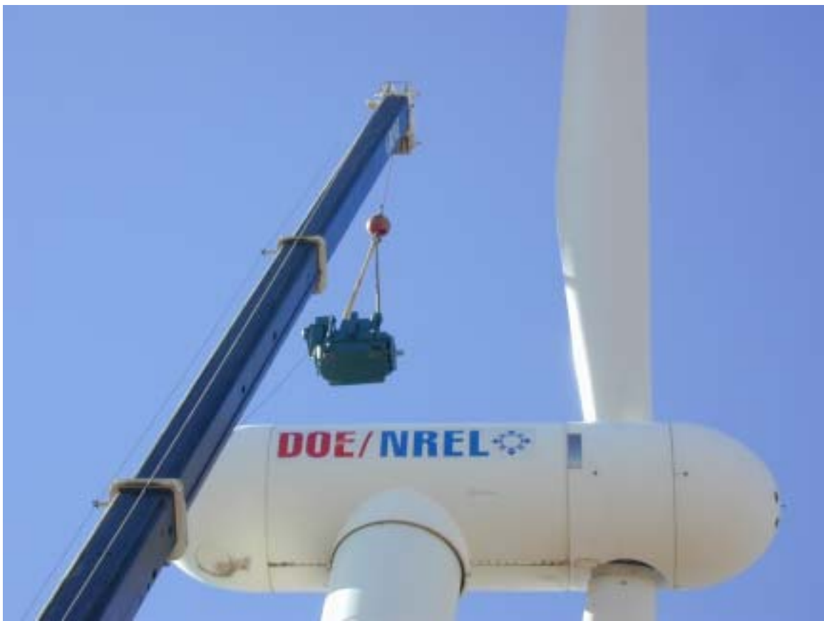
Figure 7 – New CART induction generator being installed
