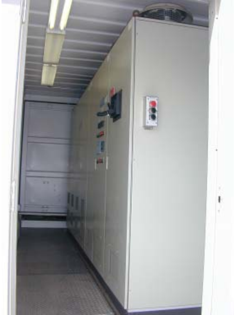
Figure 8 – Power electronics and bypass system for controlling induction generator
