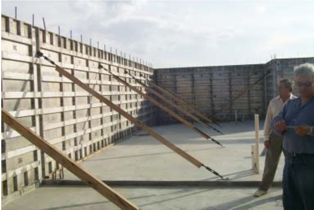
Figure 8. Modular aluminum wall forms
