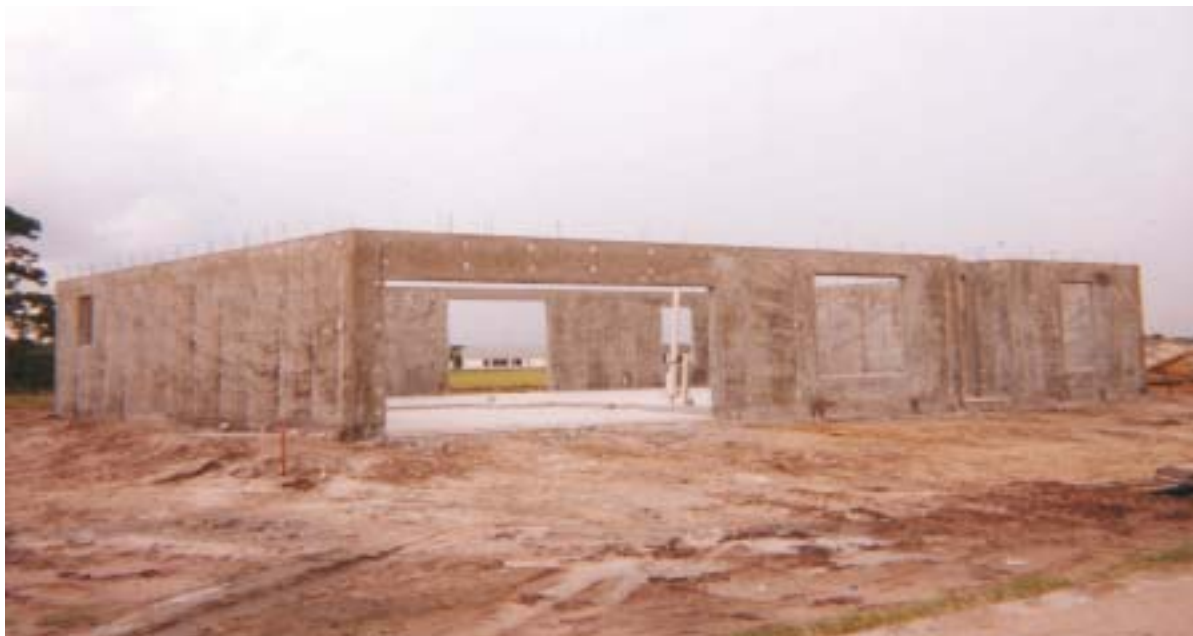
Figure 9. Concrete is poured the morning of day 2, and forms are stripped the following morning
