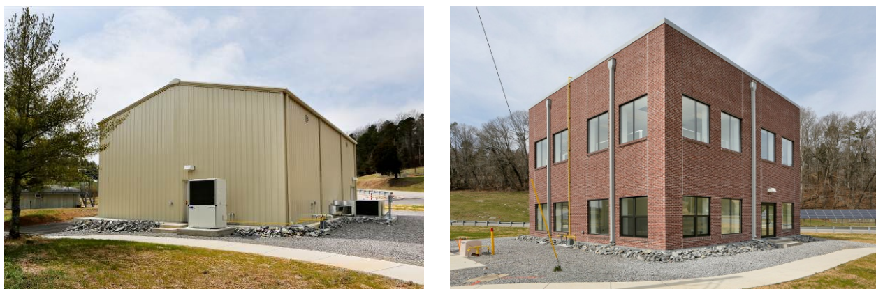
Figure 2. Flexible Research Platforms clad to emulate 1980s metal buildings (left) and office buildings from the 10-county Greater Philadelphia region (right).
