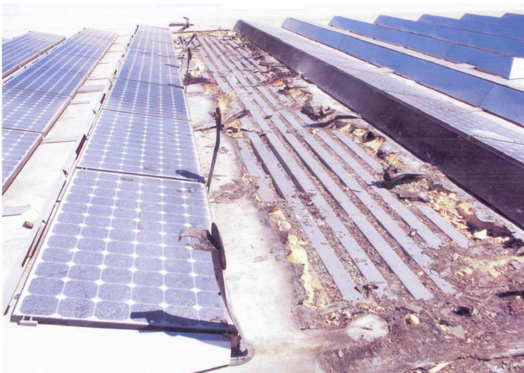
Figure 1. Aftermath of a rooftop PV fire in Bakersfield, California 2 . Photo courtesy of Pete Jackson.
