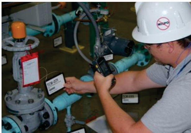
Figure 6. Operator at Catawba Nuclear Station using hand-held technology for component identification
