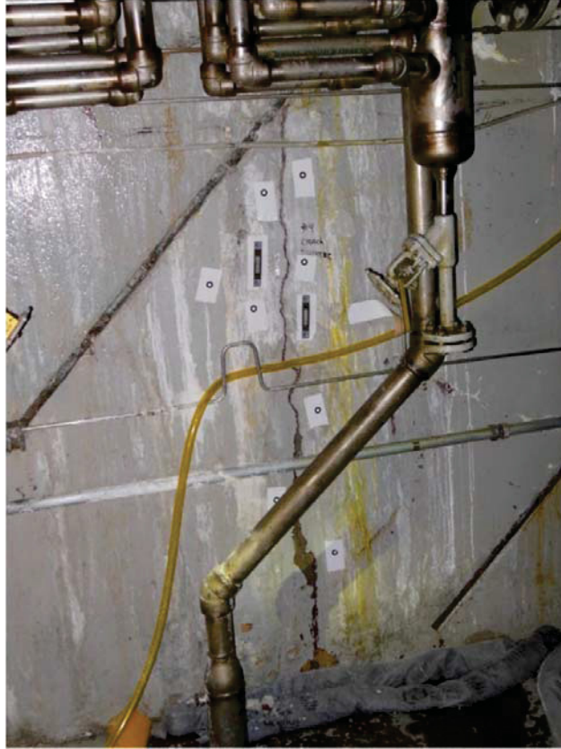
Figure 7. Example of crack monitoring.
