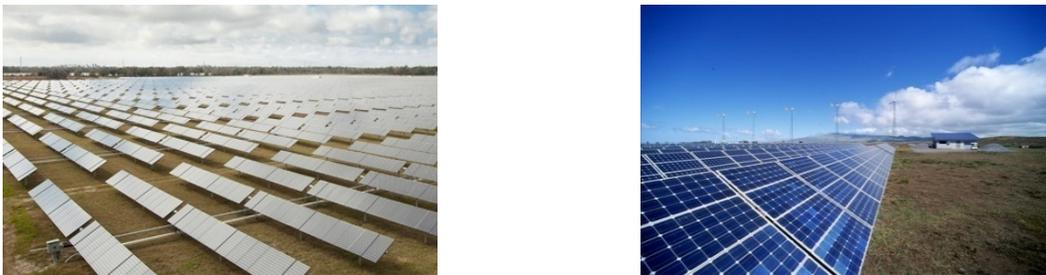
**Figure 3. Mono- and multi-crystalline solar panels. Photos from (left) SunPower Corporation, NREL 23816 and (right) SunPower, NREL 13823**
