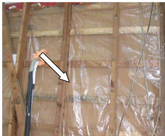
Figure 9. Wall cavity in New York where an interior vapor barrier is present.
