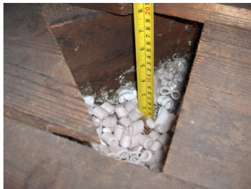
Figure 19. Packing peanuts used as insulation.
