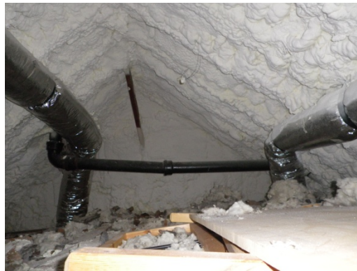
Figure 7. Open-cell spray foam on the roofline and gables.
