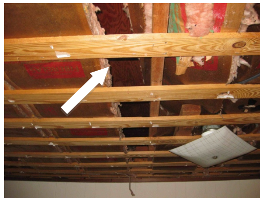
Figure 47. Ceiling insulation in the addition of South Carolina. The arrow in the figure highlights gaps in the insulation where the ceiling was not insulated from the attic air.
