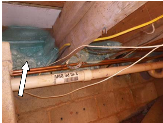
Figure 77. R-5 of closed-cell insulation sprayed on the band joist
