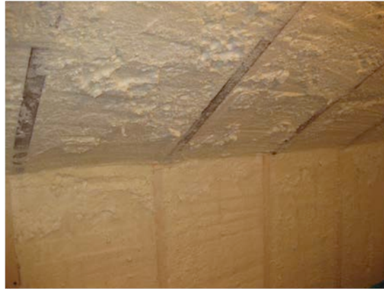
Figure 75. Photograph of open-cell spray foam in the wall cavities and ceiling rafters
