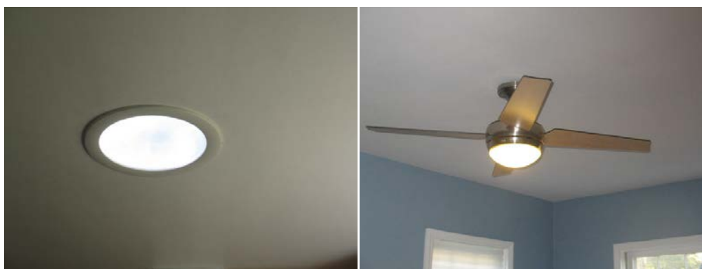
Figure 87. Sun tunnel (left) and ENERGY STAR ceiling fan (right)
