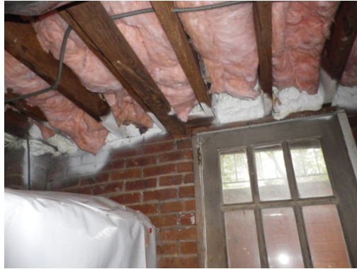
Figure 40. Fiberglass batts reinstalled in the crawlspace after air sealing
