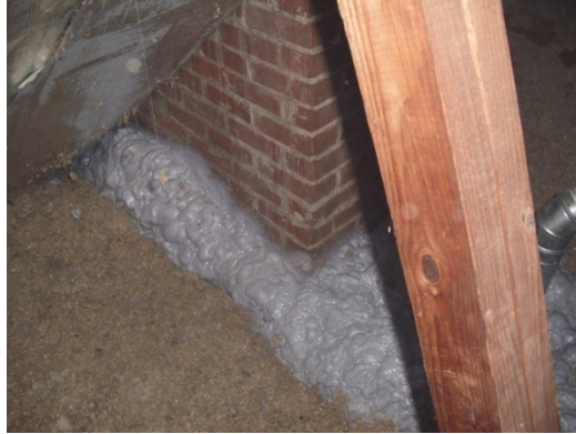
Figure 83. Spray foam insulation applied around the fireplace chase.
