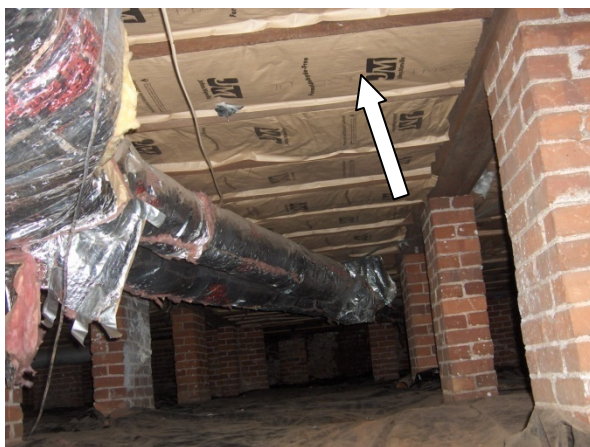
Figure 22. Photograph of the R-13 batts installed in crawlspace ceiling.
