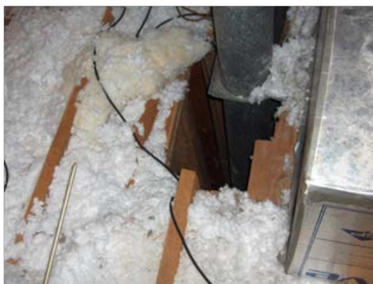
Figure 64. Open furnace chase in attic.
