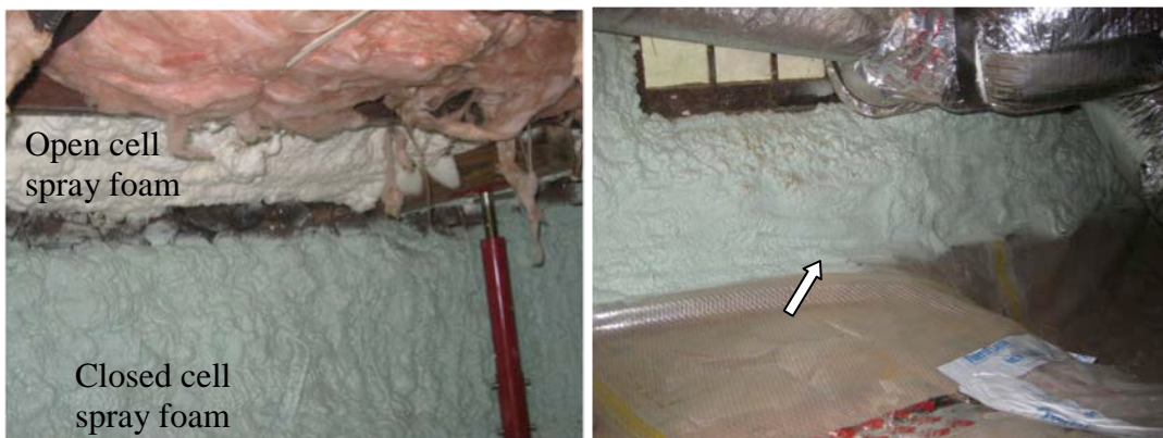
Figure 33. Crawlspace sealing and vapor barrier installation. The arrow in the picture on the right highlights the open-cell spray foam applied over the vapor barrier.
