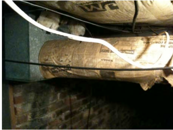
Figure 48. Ducts with newspaper used as insulation
