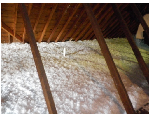
Figure 24. Blown fiberglass insulation applied in the attic ceiling (R-38).
