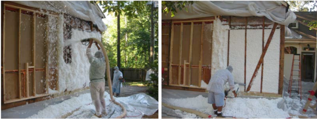
Figure 10. Spider insulation blown into the exposed cavities.
