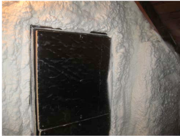
Figure 32. Insulation applied on the attic knee wall and the attic access door.
