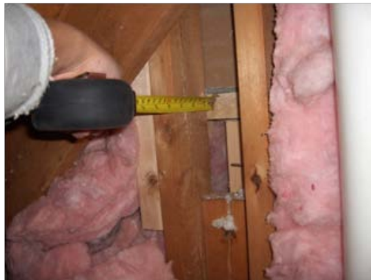
Figure 62. Void in attic knee walls
