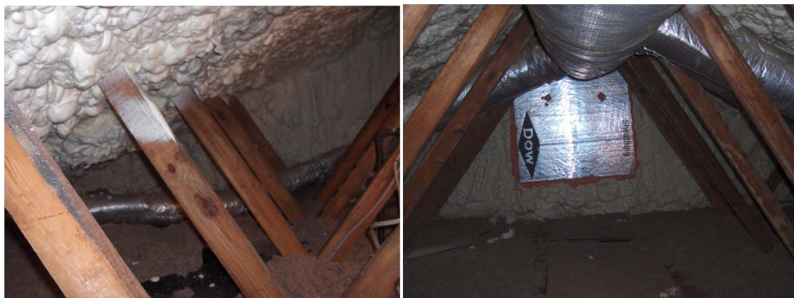
Figure 56. Open cell spray foam applied in the roofline and gables
