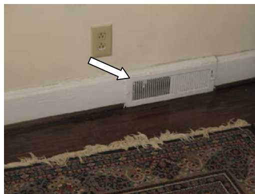
Figure 14. Duct register located in an interior wall.
