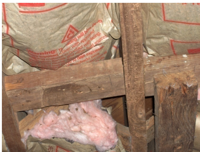
Figure 38. R-13 insulation installed in a manner inconsistent with recommended approaches.
