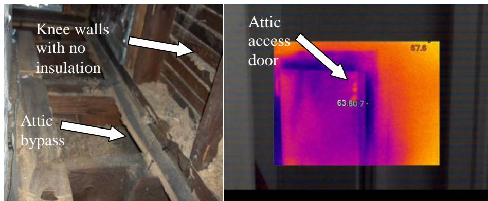
Figure 29. Attic bypasses. On the right is a thermal image of the attic access door. The blue color in the image shows attic air infiltration into the living space.
