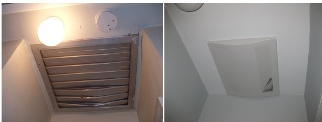
Figure 86. Spot energy recovery ventilator is shown in the image on the right. The initial whole-house fan is shown in the figure on the left.
