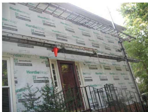
Figure 65. House wrap applied to Yellow Jackets before siding
