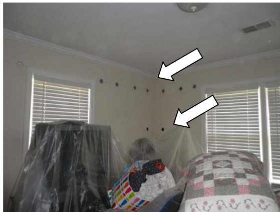
Figure 76. Holes drilled in the wall for cellulose installation
