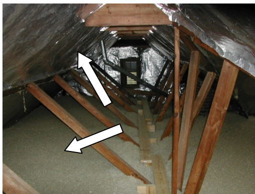
Figure 80. Photograph of the attic in Two Cities. The arrows in the figure are shown to highlight the radiant barrier on the roofline and the continuous layer of fiberglass insulation on the attic floor.
