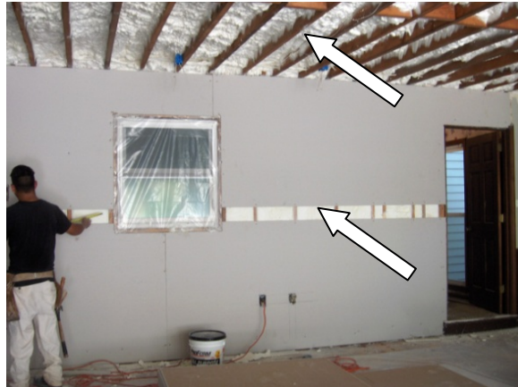
Figure 67. Insulated and sealed garage wall and ceiling. Arrows in the picture point to the spray foam in the wall cavities and in the garage ceiling.
