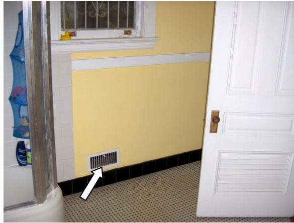
Figure 26. Photograph of supply register located in the wall.
