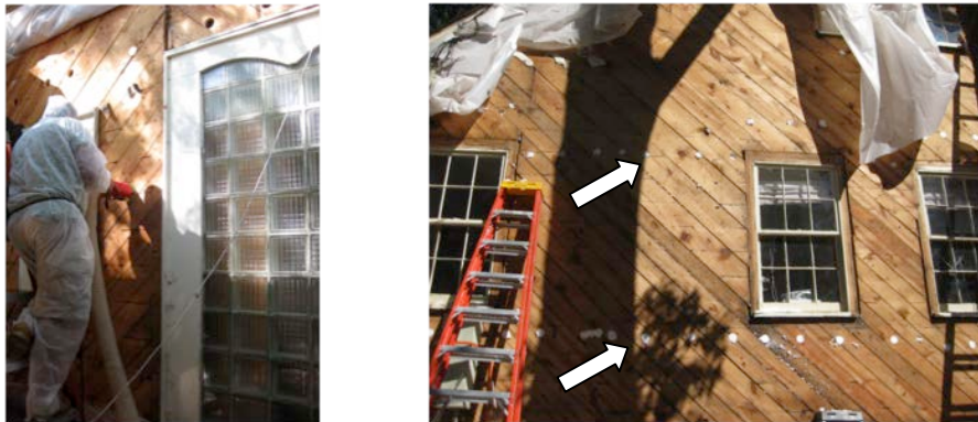
Figure 11. Photographs of the "drill-and-fill" installation of fiberglass insulation into the cavity walls. Image on the left shows the installer blowing fiberglass into the cavity. Two holes in each cavity can be seen in the image on the right.
