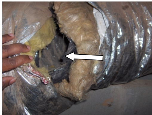
Figure 31. Disconnected ducts in the crawlspace
