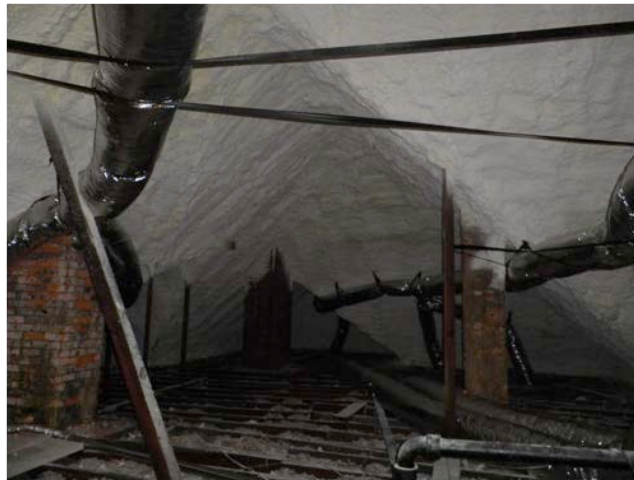
Figure 49. Photograph of attic after open-cell spray foam has been applied to the roofline
