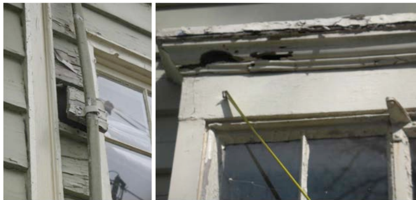
Figure 5. Photographs show examples of places in the exterior siding where rotting has occurred.
