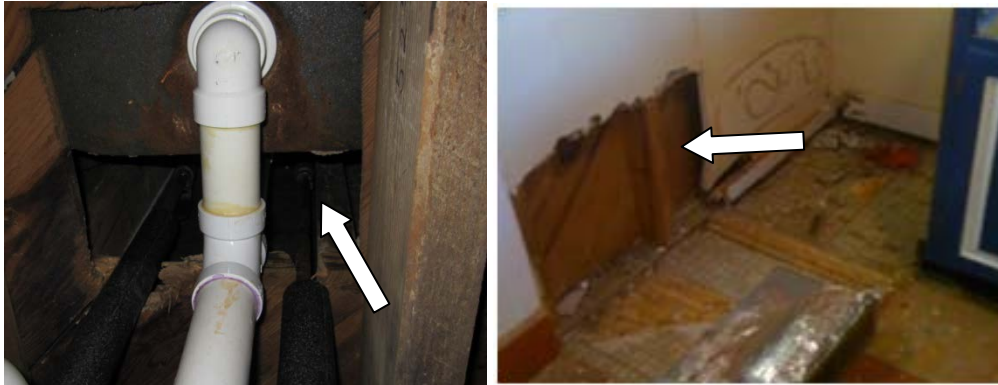
Figure 82. Infiltration pathways found in Two Cities. The photograph on the left shows an open plumbing access underneath the tub. The image on the right shows a hole in the kitchen wall behind a cabinet.
