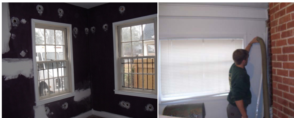
Figure 84. Drill and fill of cellulose insulation in the exterior wall cavities.
