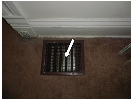
Figure 51. Capped floor register
