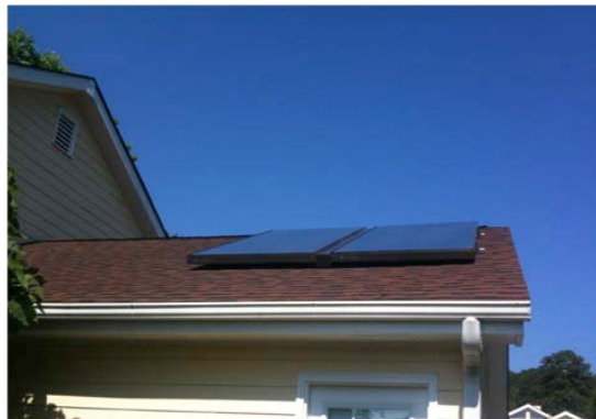
Figure 58. Solar thermal hot water panels installed on the garage roof.
