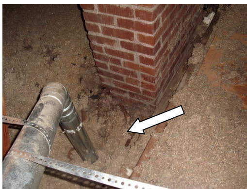
Figure 81. Open chase near the fireplace chimney and water heater flue.
