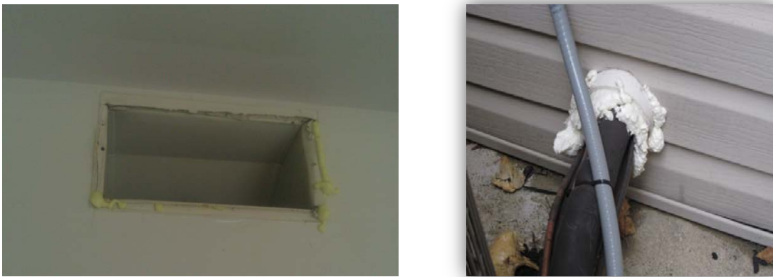
Figure 6. Air sealing of duct register boot and an HVAC penetration
