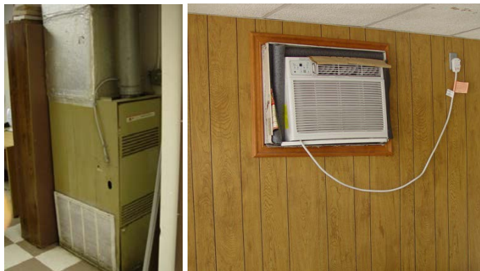
Figure 5. Natural gas furnace (left); window AC unit, fitted into rough opening with cardboard and foam (right)
