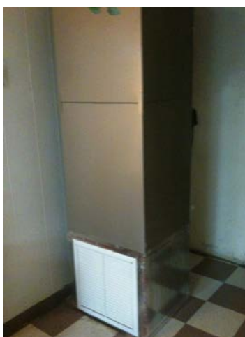
Figure 14. Post-retrofit ground floor, SEER 15 heat pump AHU
