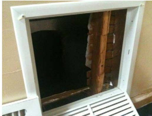
Figure 13. Post-retrofit, researchers observed an airflow pathway from a large open wall cavity between the AHU and the filter grille
