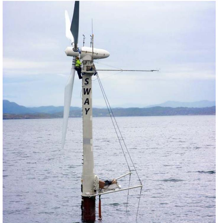
In 2012, NREL sent staff to SWAY's offshore wind project in Norway to install scientific equipment on the seabed and the prototype to collect data that will help validate NREL's computer model. *Photo by Robb Wallen, NREL/PIX 22134*
