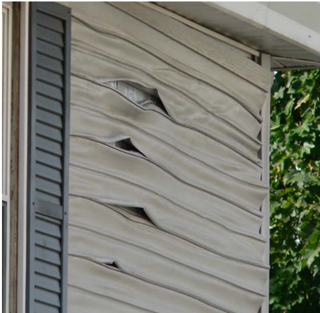
Figure 1a. Vinyl siding with extreme permanent distortion
