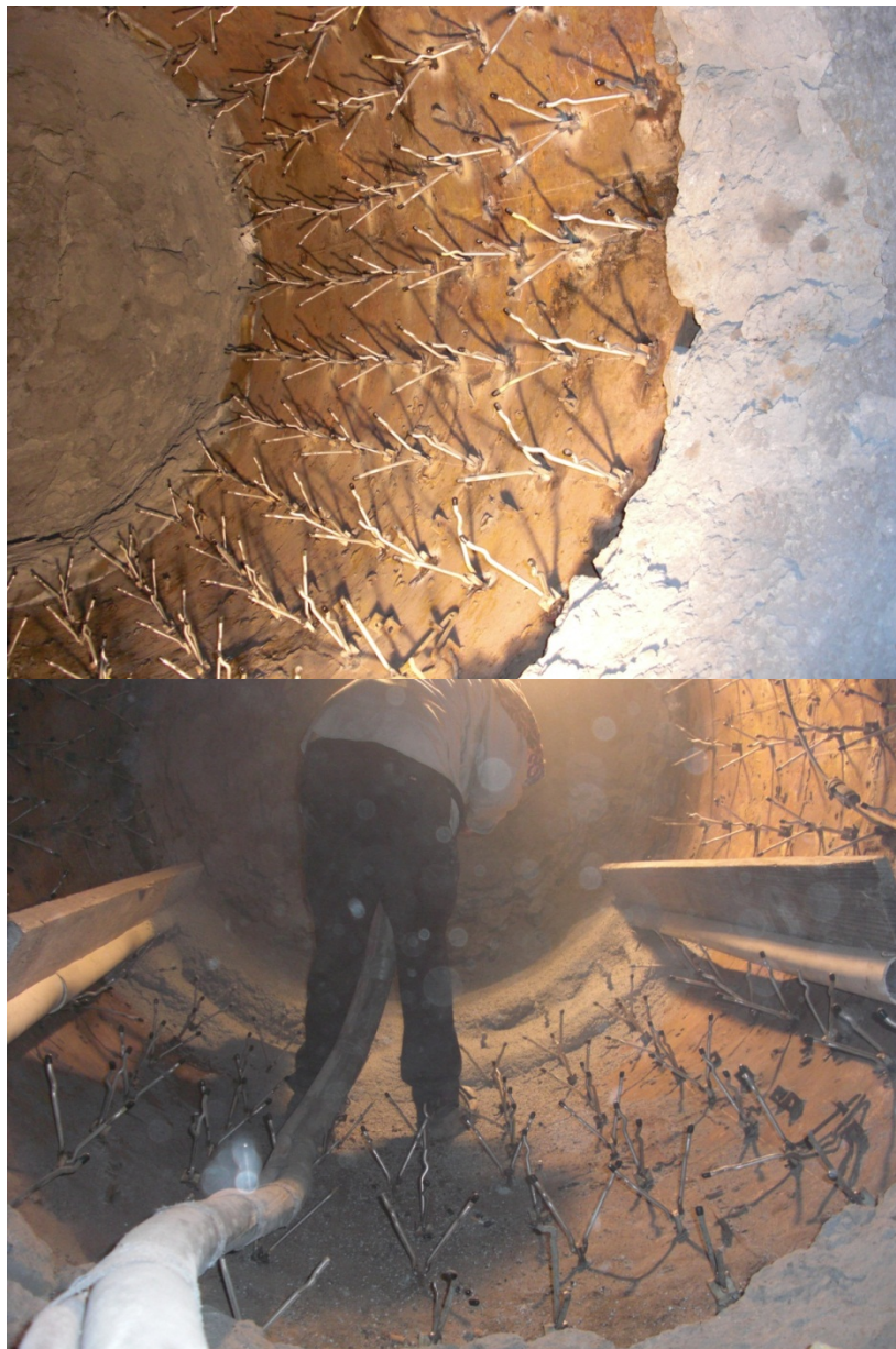
Figure 104. Aluminum Rotary Dross Furnace at Newco Metals (Bedford, IN) Before and During Installation of Developed Aluminum Furnace Refractory
