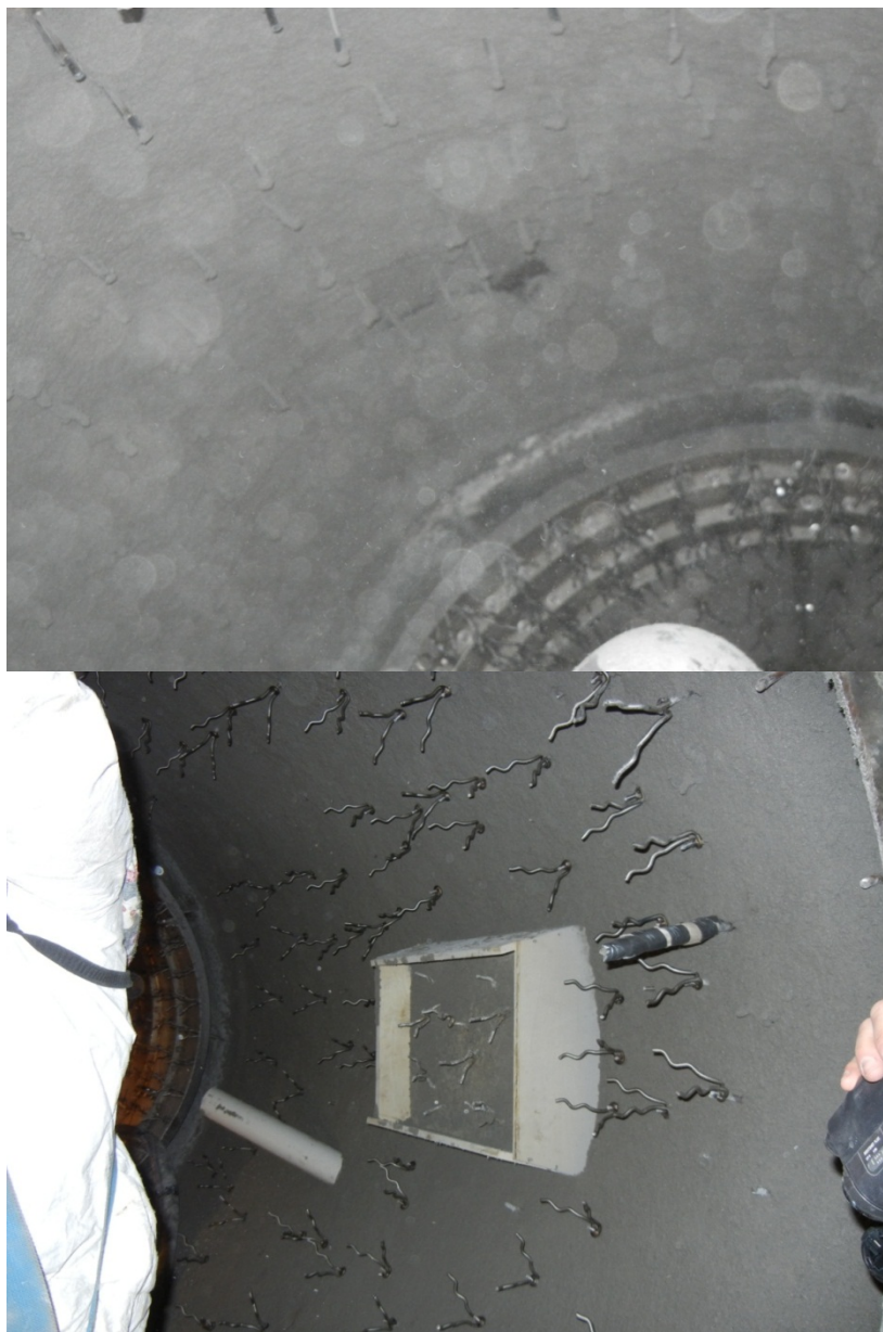
Figure 109. Installed Insulshot Lightweight Back-up Refractory at Tate & Lyle (Lafayette, IN)
