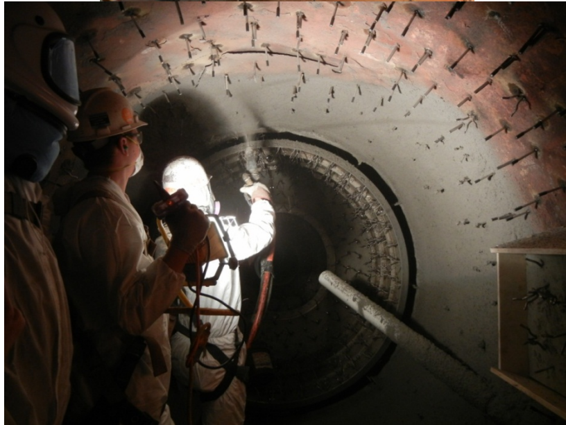
Figure 108. Installation of Light Weight Refractory in Combustion Zone of Dryer
