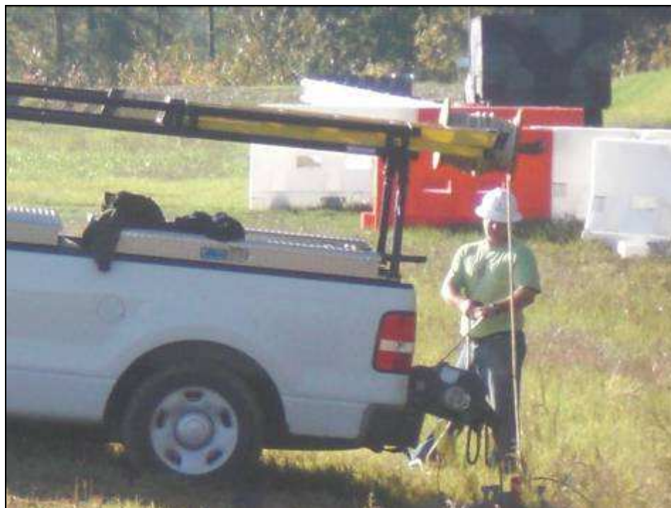
Figure 45: Winching Copper Cable Through Innerduct
