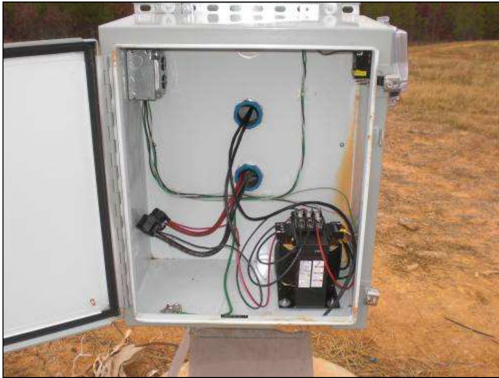
Figure 49: Copper terminations at Base of Pole
