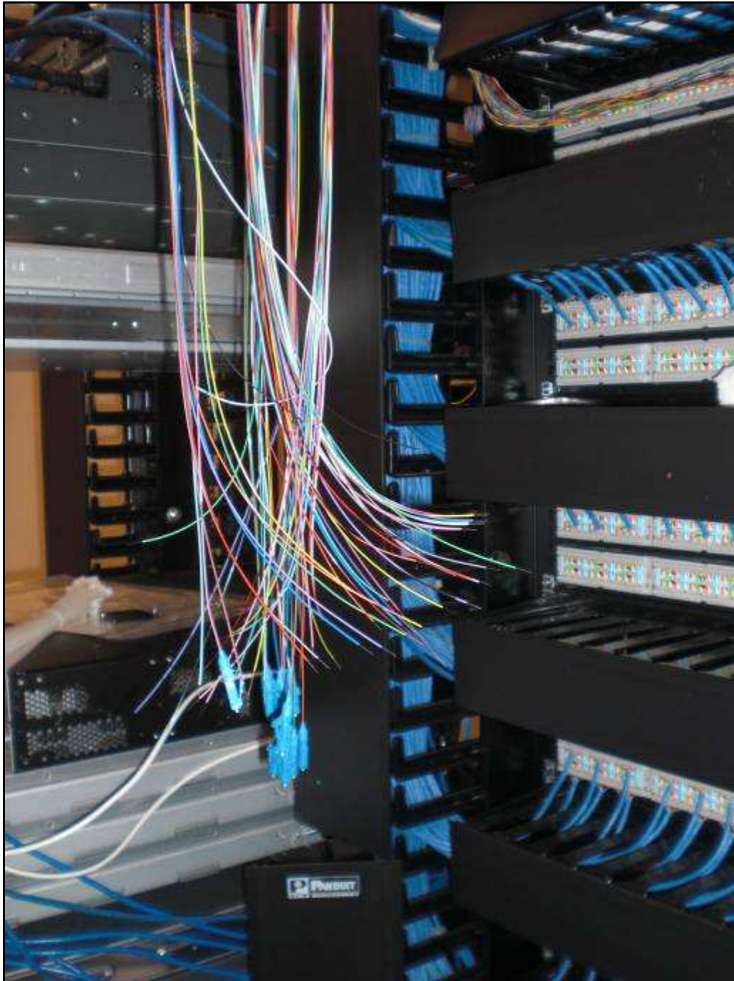
Figure 51: Site Fibers Terminating in IT Room
