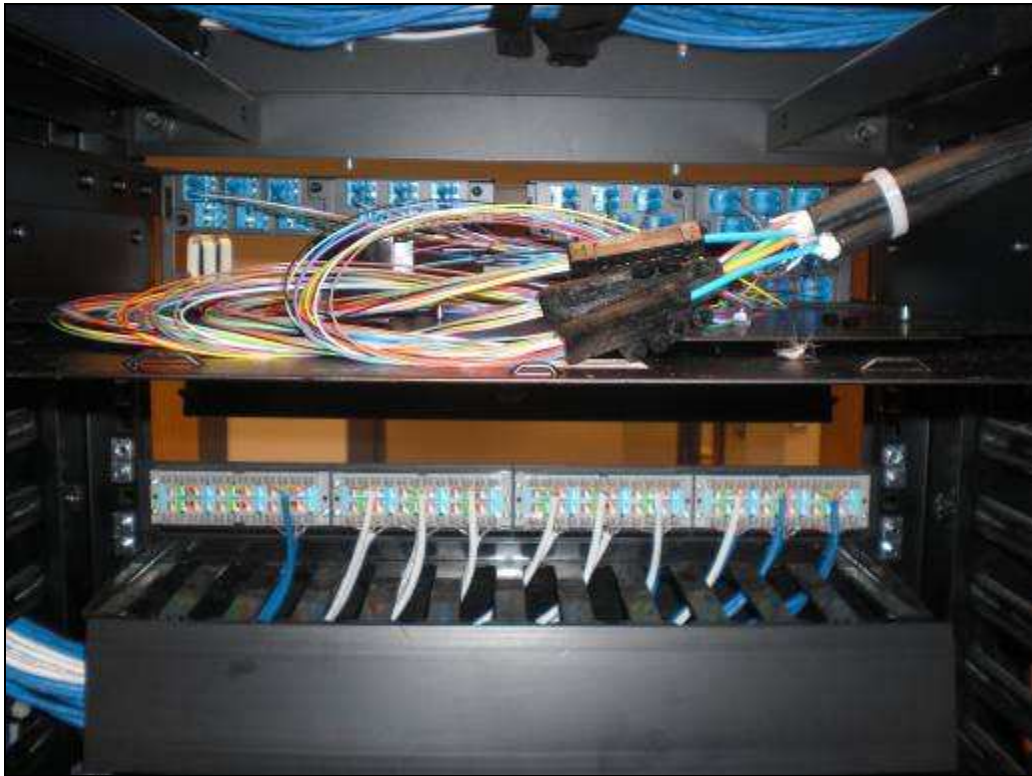
Figure 52: Fibers Terminated at Rear of Switch
