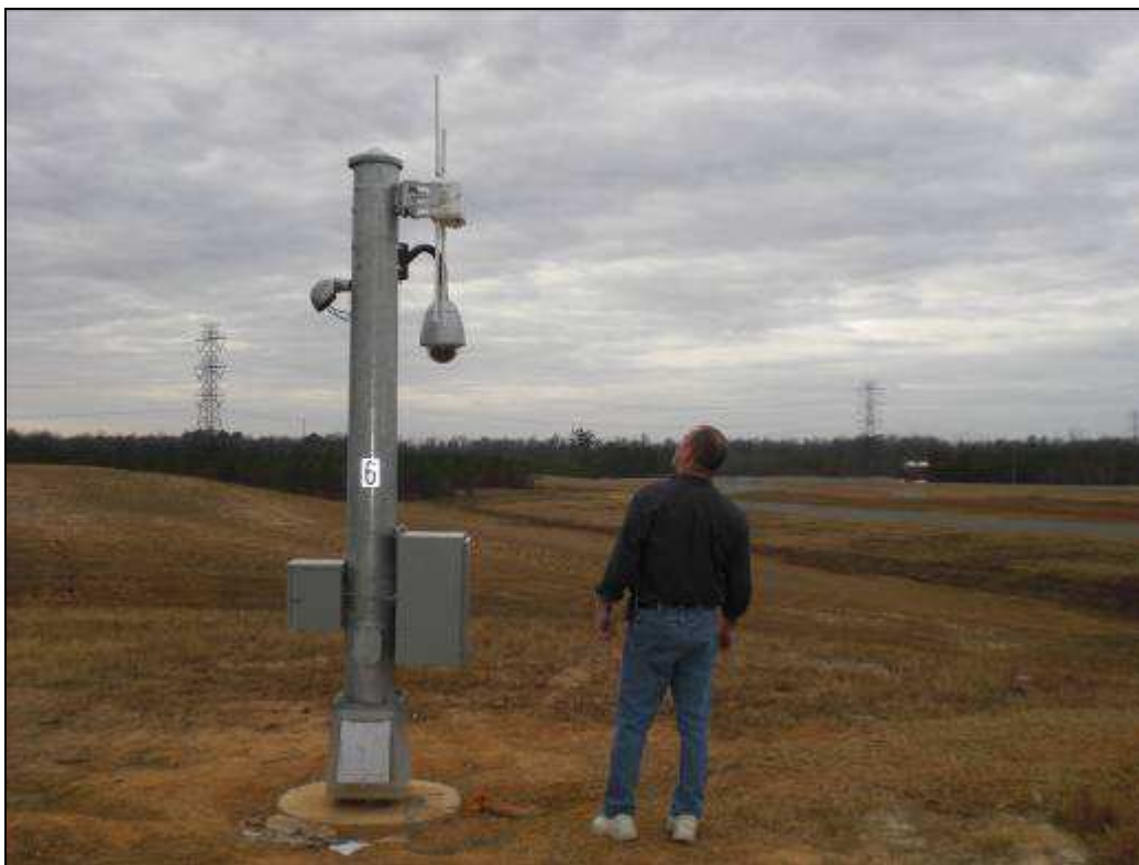
Figure 50: Pole Installation Complete (pole #6 is only 10ft tall due to location on 25ft hill)
