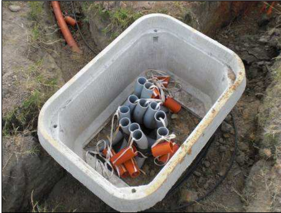
Figure 42: Pull Boxes Located Across Site to Facilitate Long Pulls
