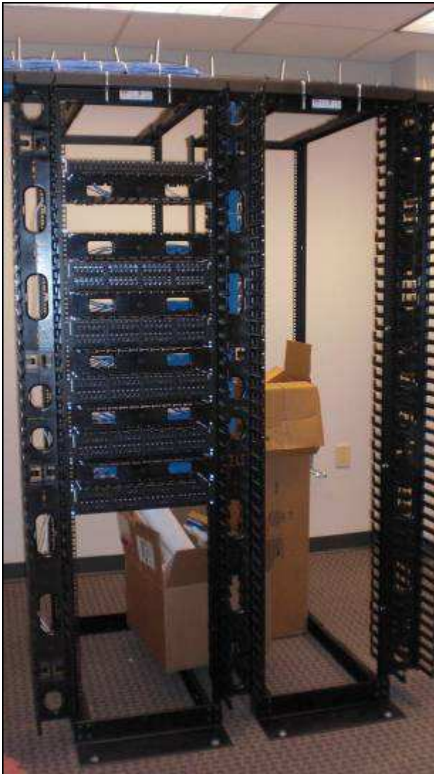
Figure 28: IT Racking System in IT Room
