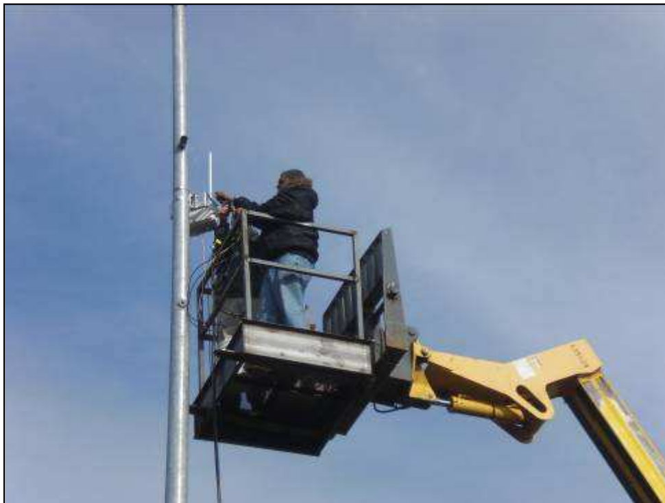
Figure 46: Camera & AP Installation on Pole # 2
