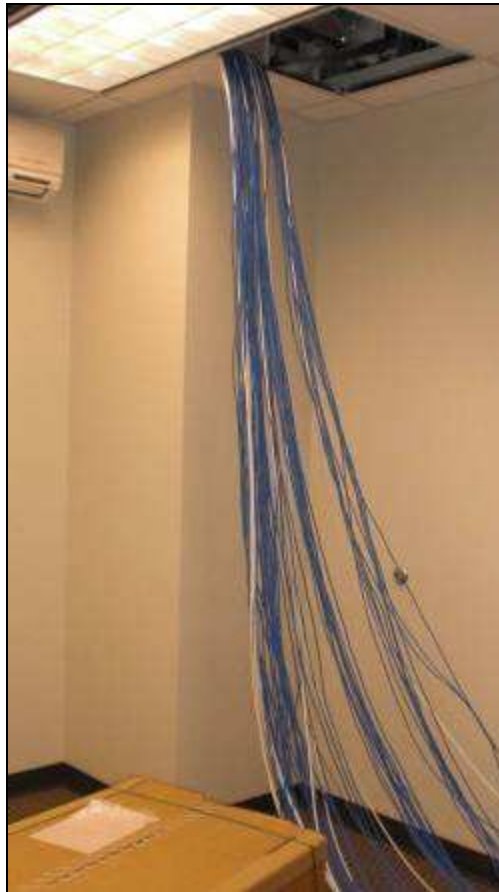
Figure 26: Cable Pulls Enter IT Room
