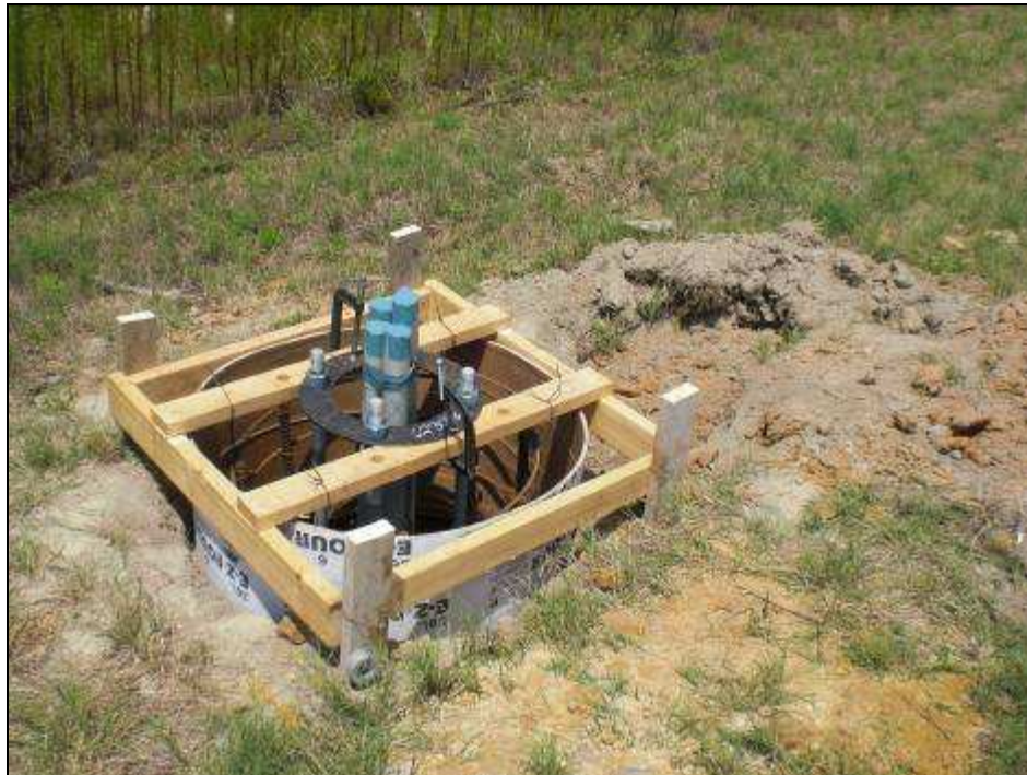
Figure 36: Tower Base Ready for Concrete Pouring
