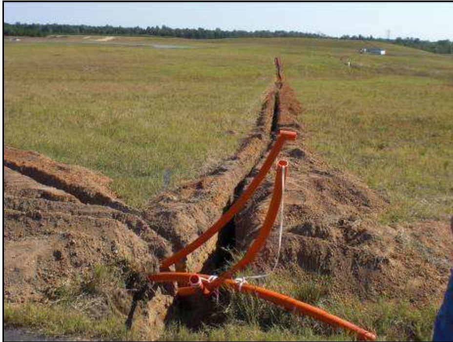
Figure 40: Site Trenching – Innerduct in Place (awaiting copper pulls)
