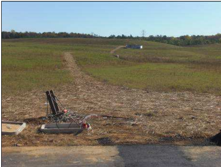
Figure 43: Filled & Seeded Trenches
