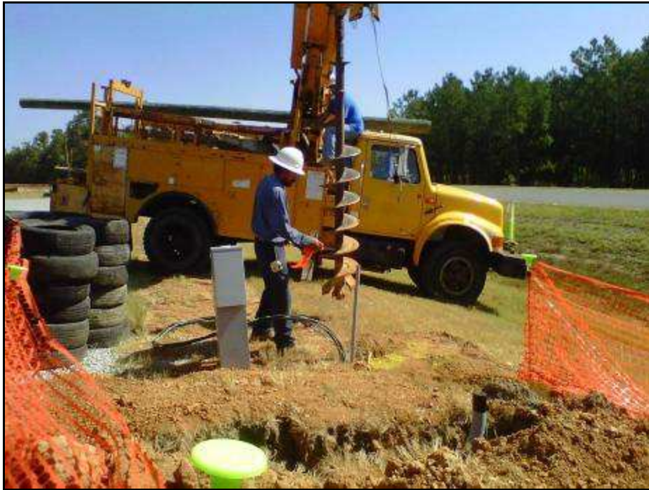
Figure 11: Pole Installation at Paddock
