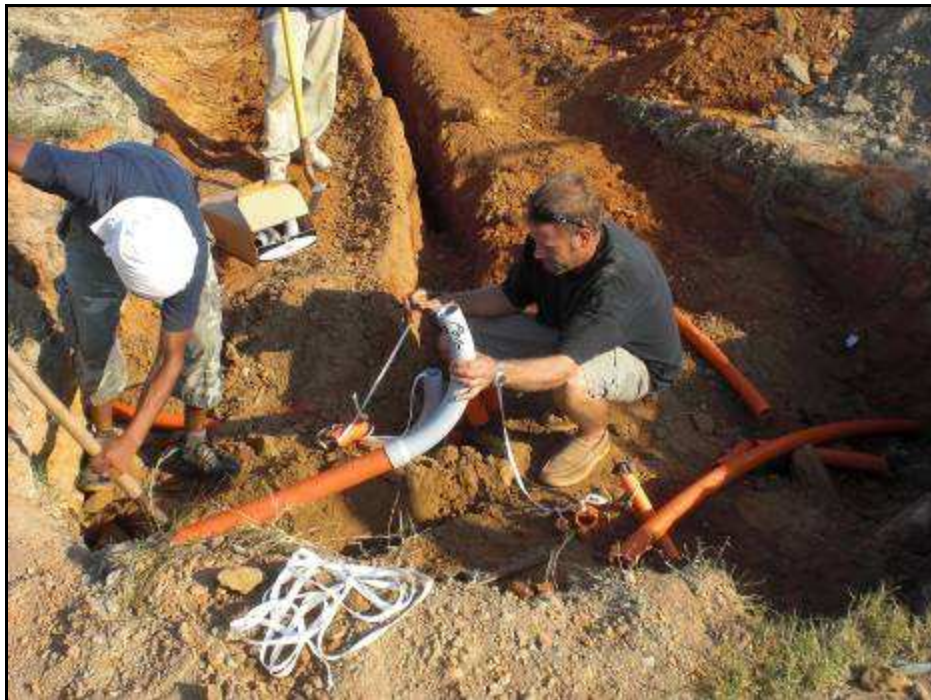
Figure 41: Pull Lines Ready for Copper Pulls
