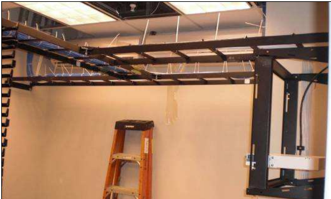
Figure 27: IT Room Overhead Cable Ladder Tray Installation
