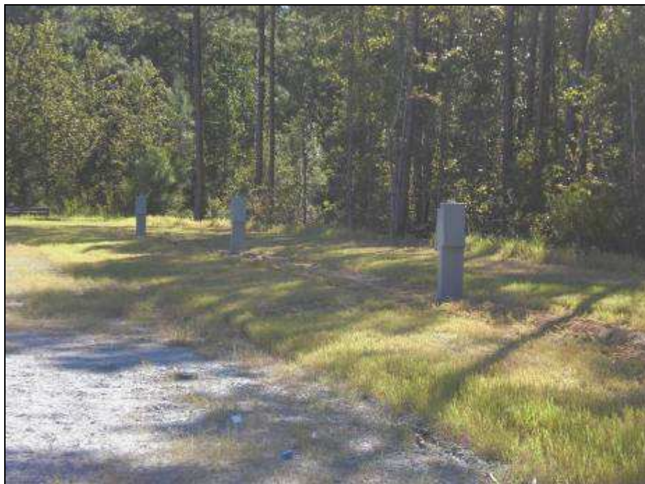
Figures 10: Paddock Area Electrical Outlets Installed (31 in total)
