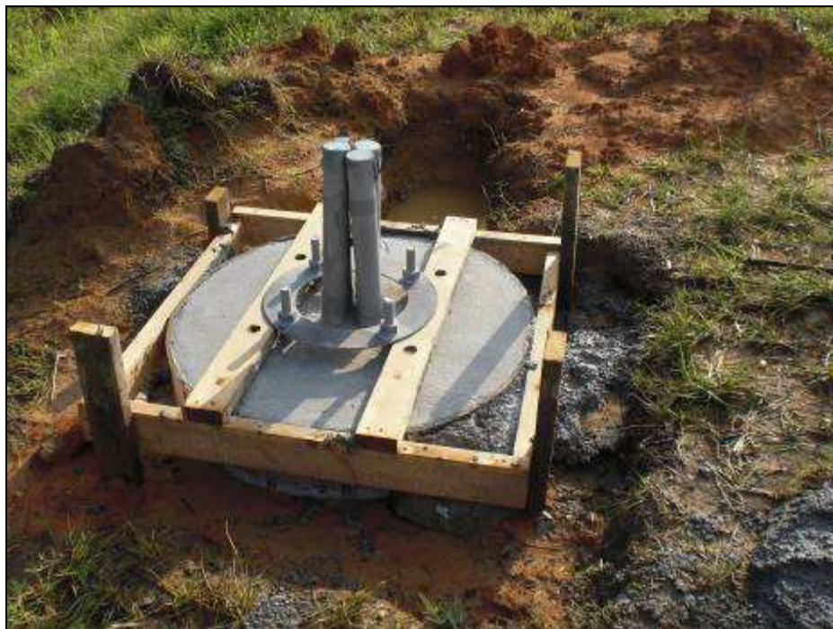
Figure 37: Tower Base Completed
