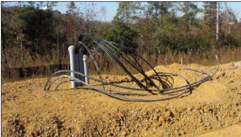
Figure 4: Power Termination at Transformer Location
