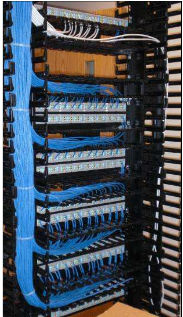
Figure 29: Cables Installed on Reverse Side of Racks
