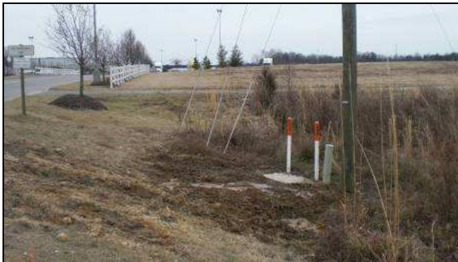
Figure 21: ISP Fiber Markers at Head of NCCAR Access Road
