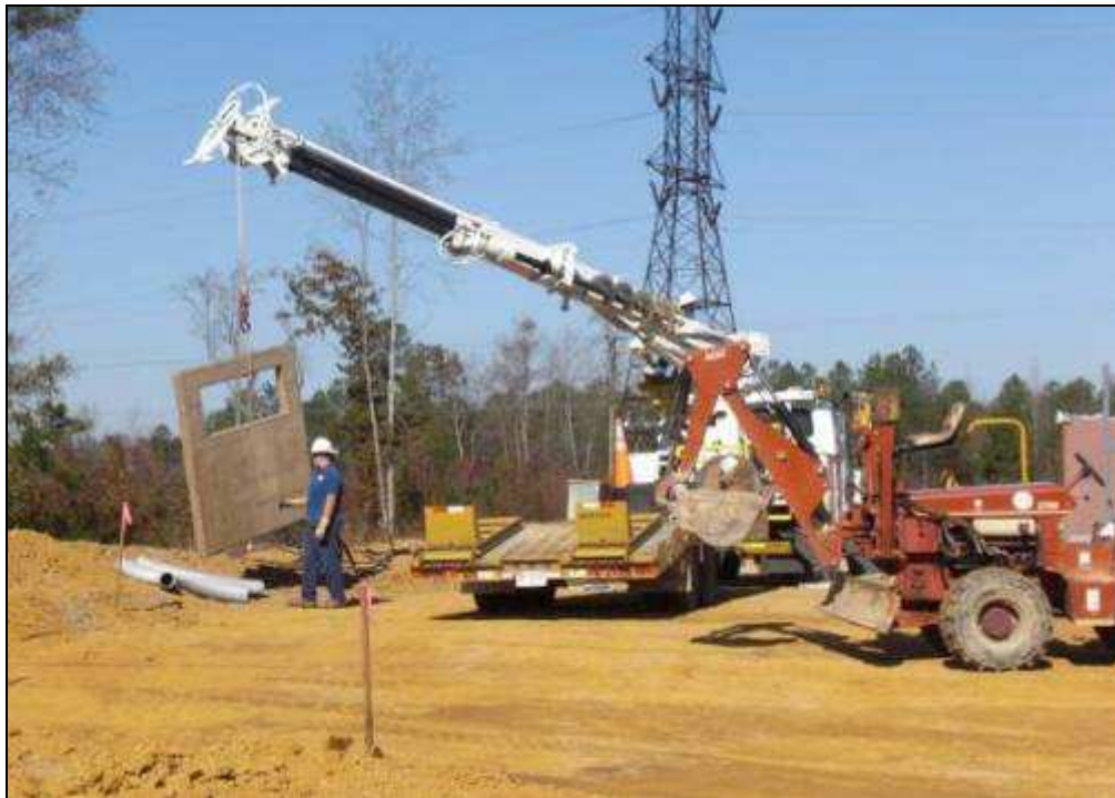
Figure 5: Transformer Base Plate Installation at Operations Building
