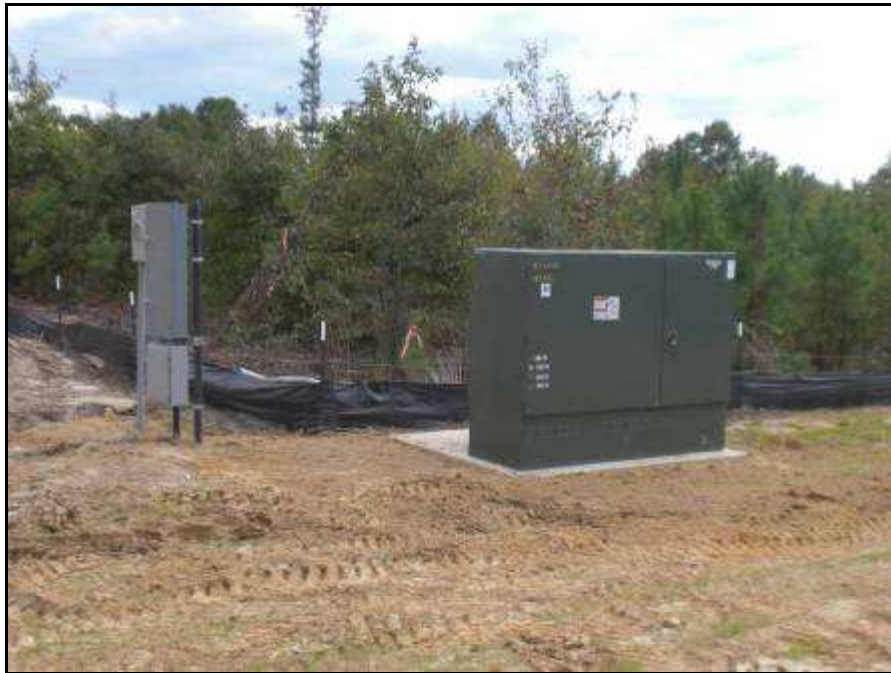
Figure 15: Transformer installation Complete (plus MDP for poles & future building)
