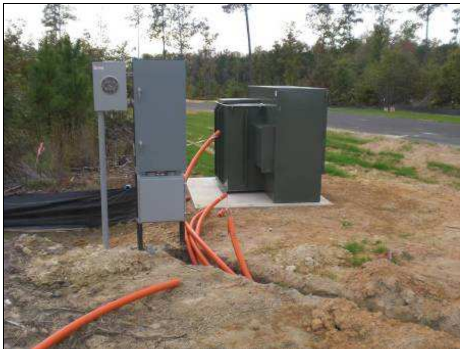
Figure 14: Innerduct Trenches Leading to Poles
