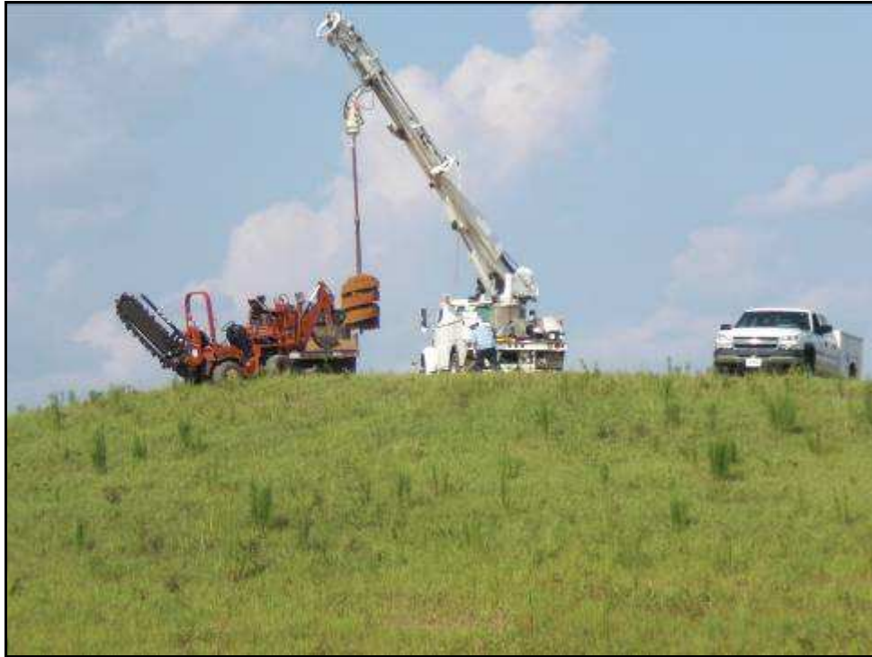
Figure 34: Boring of Tower Base
