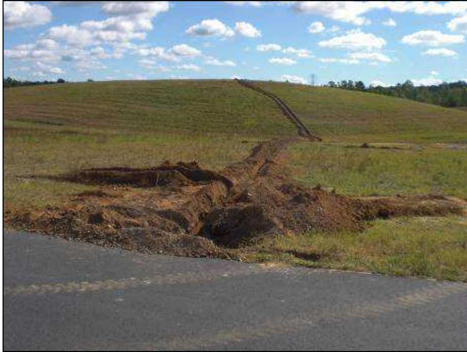
Figure 38: Site Trenching (awaiting copper & fiber)
