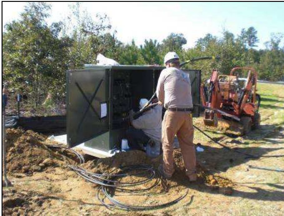
Figures 13: Installation of Transformer at Track Location
