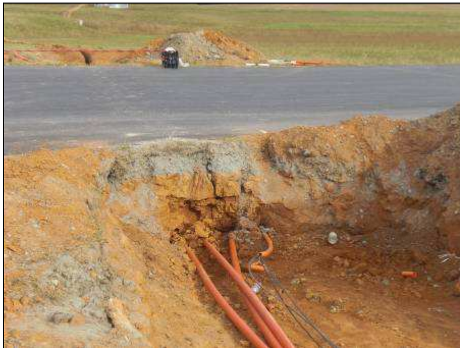
Figure 39: Directional Bores Under Test Track
