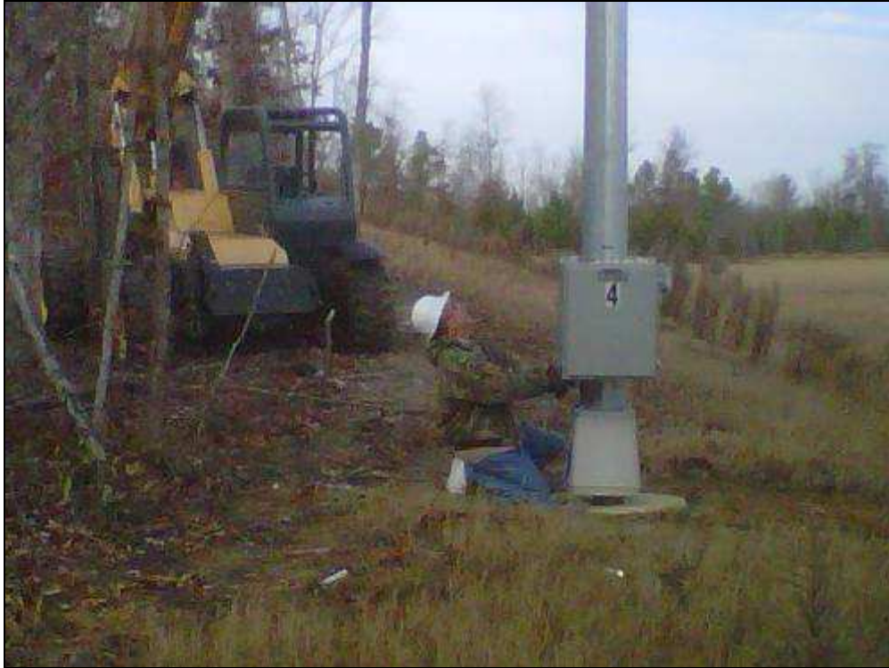
Figure 48: Fiber & Copper Connections at Pole Base
