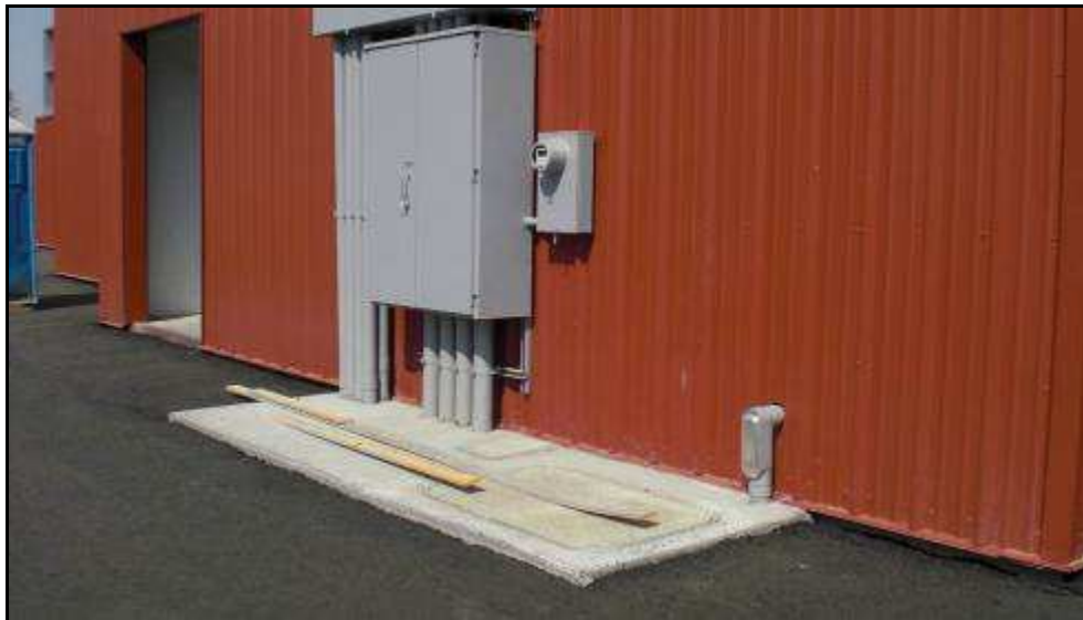
Figure 8: Electrical Supply & Telecoms into Rear of Operations Building
