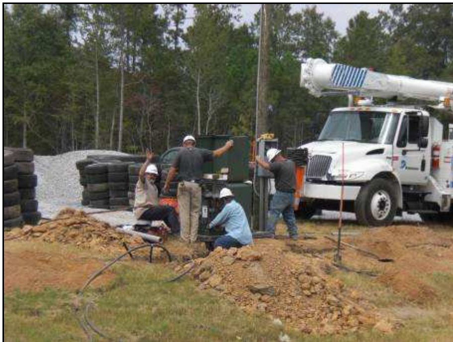
Figure 12: Power Transformer Installation at Paddock
