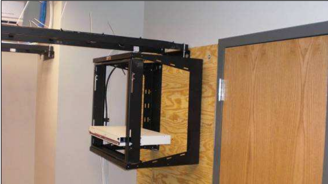
Figure 24: ISP Wall Rack in IT Room (Operations Building)
