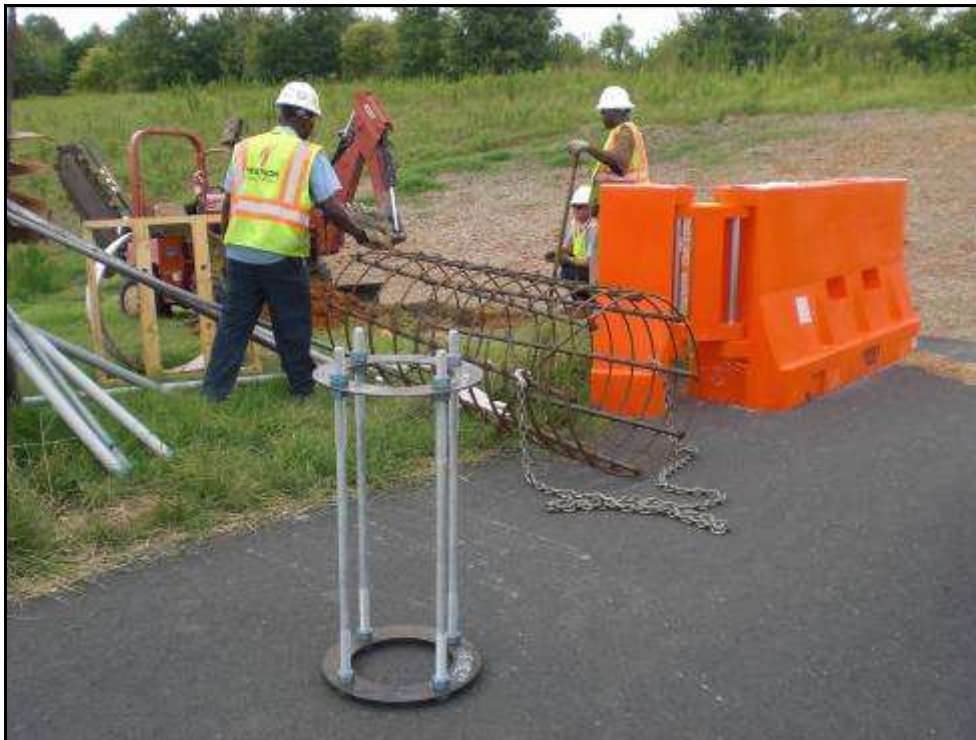
Figure 35: Tower Base Foundation Re-Bar
