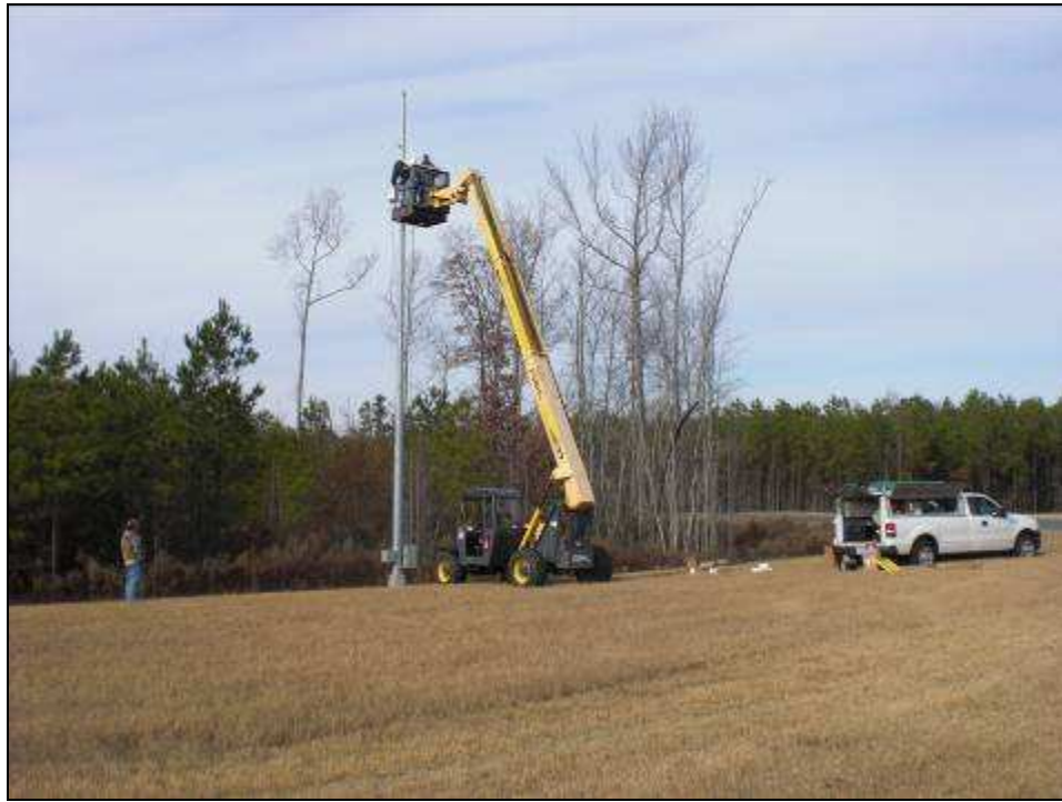
Figure 46: Camera & AP Installation on Pole # 2
