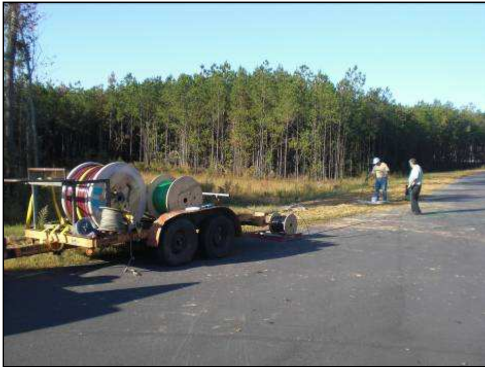
Figure 44: Copper Cable Pull
