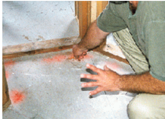
Figure 19. Paint tags alerting crews to the location of the proposed chase.
