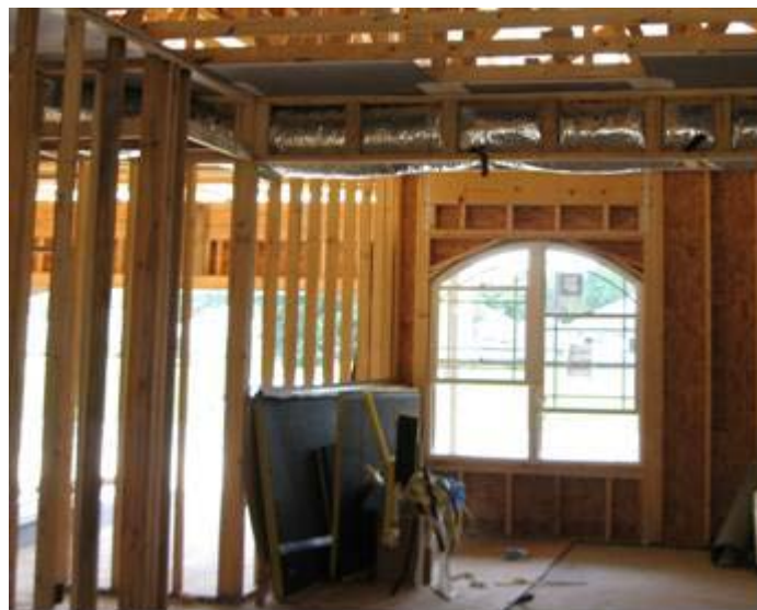
Figure 28. Chase sides and bottom installed.
