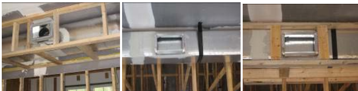
Figure 29-31. (Left to right) Connecting flex duct to a trunk line for a supply run-out results in a wide chase. Instead, a supply outlet constructed from a duct board box can be directly affixed to the trunk. This permits construction of a much narrower chase.
