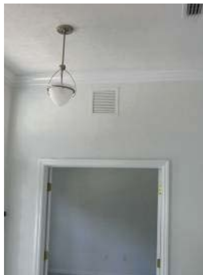
Figure 14. Transom return pathway, through the wall, over doorway of a master bedroom.
