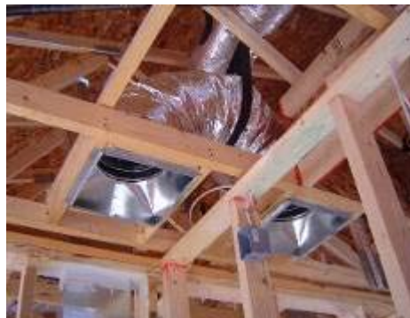
Figure 13. A jump duct through the attic. This will provide return air, over the interior wall. Note this is not an interior duct unless the attic is sealed.
