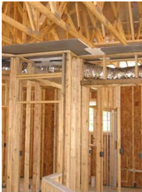
Figure 2. Fur-down chase after rough framing.
