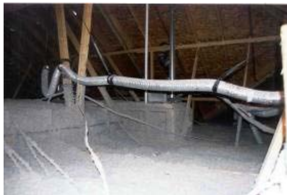
Figure 5. Poorly insulated fur-up chase sides.
