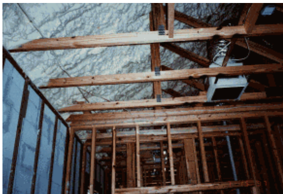
Figure 3. An unvented attic constructed by air sealing the roof deck with foam insulation. Note how the attic duct is now within the home's air and thermal barrier
