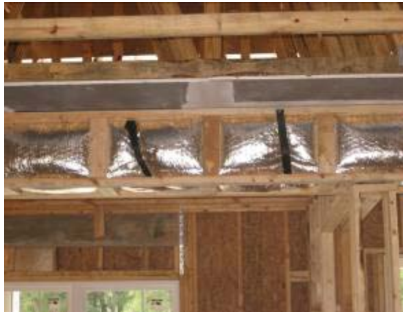
Figure 23. Finish framing for chase.
