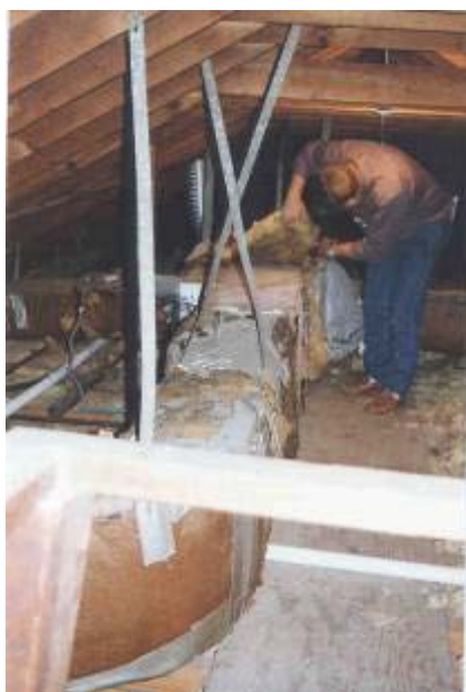
Figure 12. Air handler and duct system installed in a conventional attic. A relatively large volume of air becomes trapped in the system between runtime events, and can encounter significant heat gain/loss to the point where it can cause comfort issues when introduced into the home’s interior.
