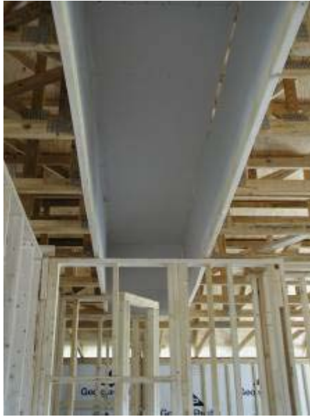
Figure 1. Fur-up chase installed after rough framing.
