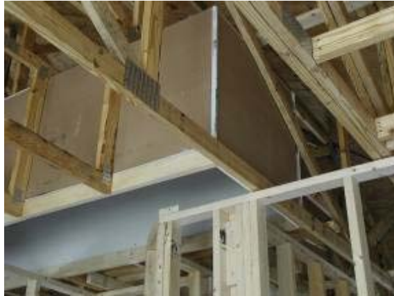
Figure 6. Modified truss work necessitated by fur-up chase.
