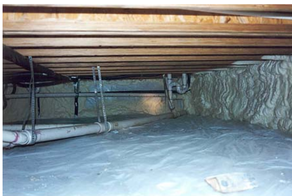
Figure 4. A sealed crawlspace by air sealing the foundation walls with foam insulation.
