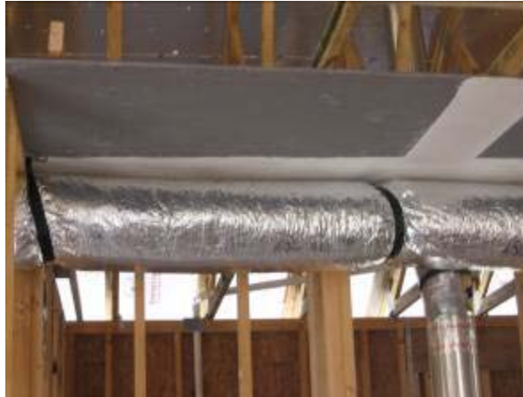
Figure 22. Duct work strapped in place prior to finishing the framing of the chase.
