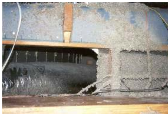
Figure 7. Fur-up chase deliberately used for wiring runs. Also note the poor overall insulation of the chase.
