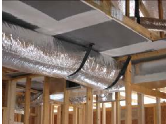
Figure 27. Duct work hung with 2" strapping after chase ceiling drywall installed and sealed.
