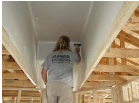
Figure 24. Air-sealing a fur-up chase.
