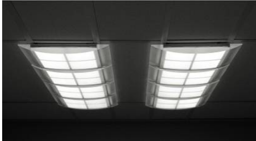
Figure 21: OLED lighting luminaires mounted in a ceiling system. Each luminaire is comprised of four 15cm x 15cm lighting panels mounted in outcoupling enhancement lenses.
