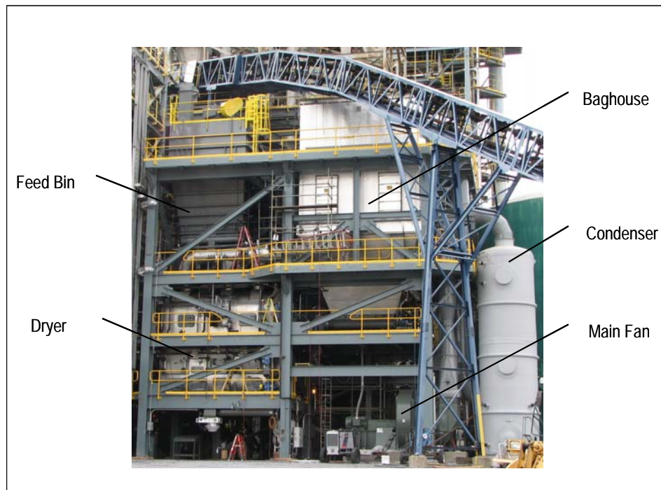
Figure 2-2. Fluid Bed Dryer System Installed at PSDF.
