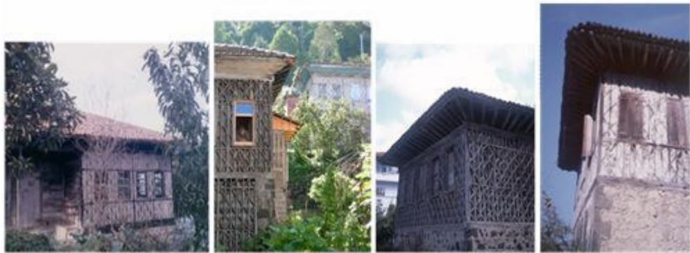
Figure 5. Examples of traditional houses built with triangular infill technique with or without infills.
