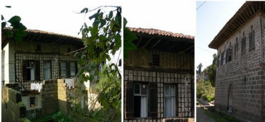
Figure 4. Examples of traditional houses built with cellular infill technique.
