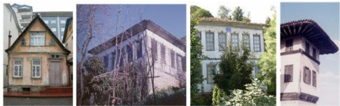
Figure 6. Terracota tile cover material and examples of veneered and fair faced eaves.
