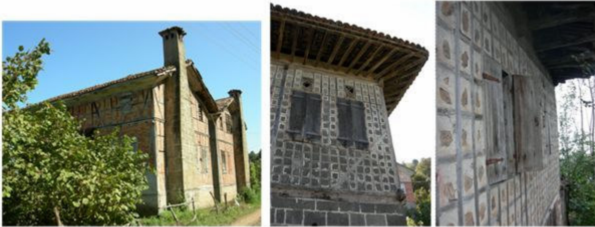
Figure 3. Examples of cellular infill systems with brick and stone fillers.
