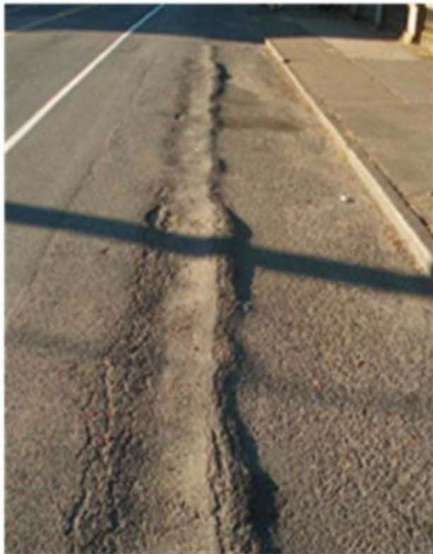
Figure 5. Permanent deformation in asphalt pavement.
