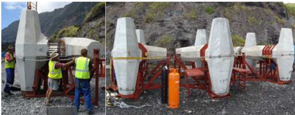
Figure 10. Stitch casting yard at Tristan da Cunha
