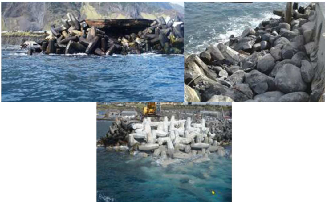
Figure 11. Stages of construction (left to right). (1) The damaged section of the Western Breakwater upon arrival of repair team; (2) the dressed armour slope; (3) completed repair – 1 April 2011.
