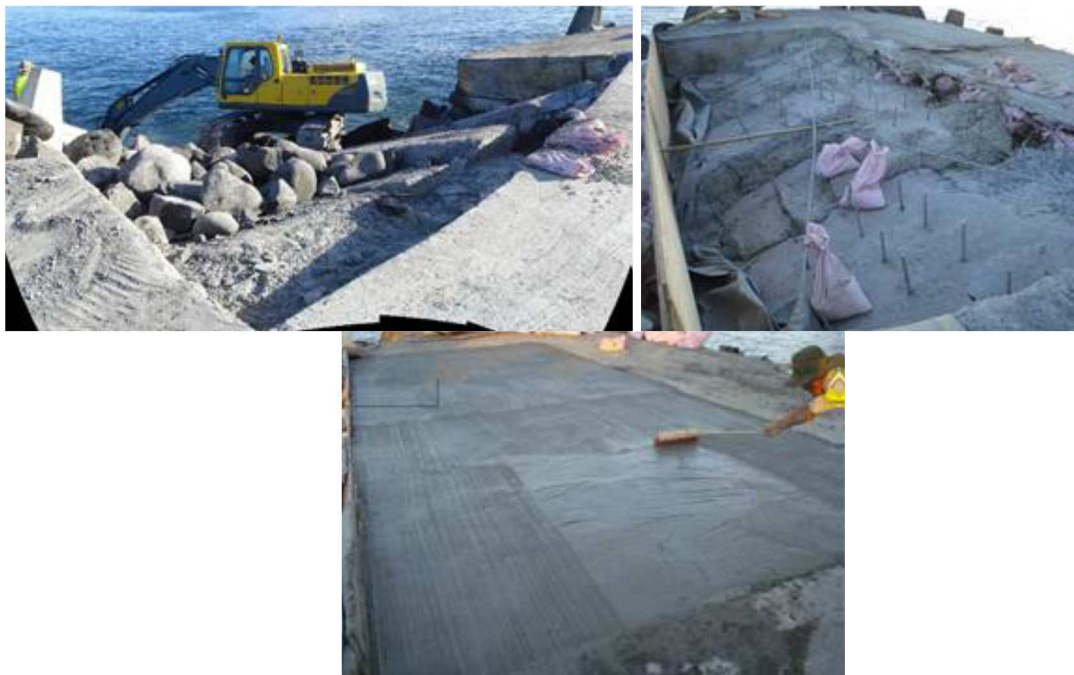
Figure 13. Stages of the concrete cap repair.
