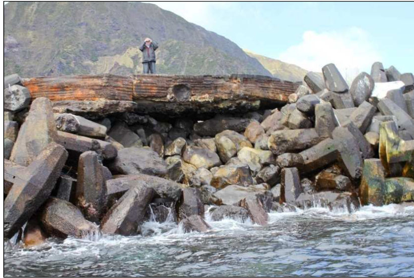
Figure 2. Photo taken 12 Sept. 2010 towards the south south-east showing the undermined deck slab and exposed core rocks near the head of the western breakwater (WSP, 2011).
