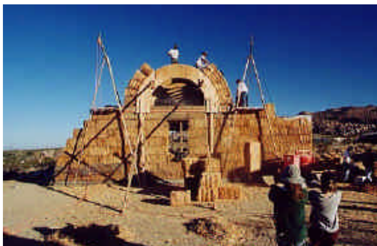
Figure 5. Straw bale load bearing wall structure, California [1]
