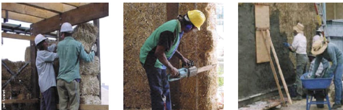
Figure 6. Technology for building a frame structure with straw bale non-load bearing walls [5]
