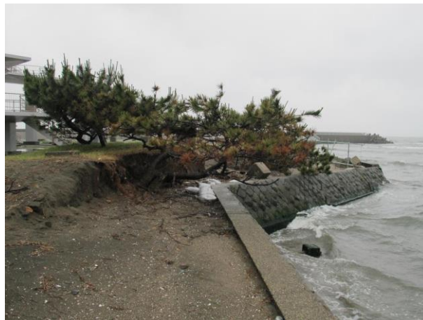
Figure 10. Erosion behind seawall and scarp formation.
