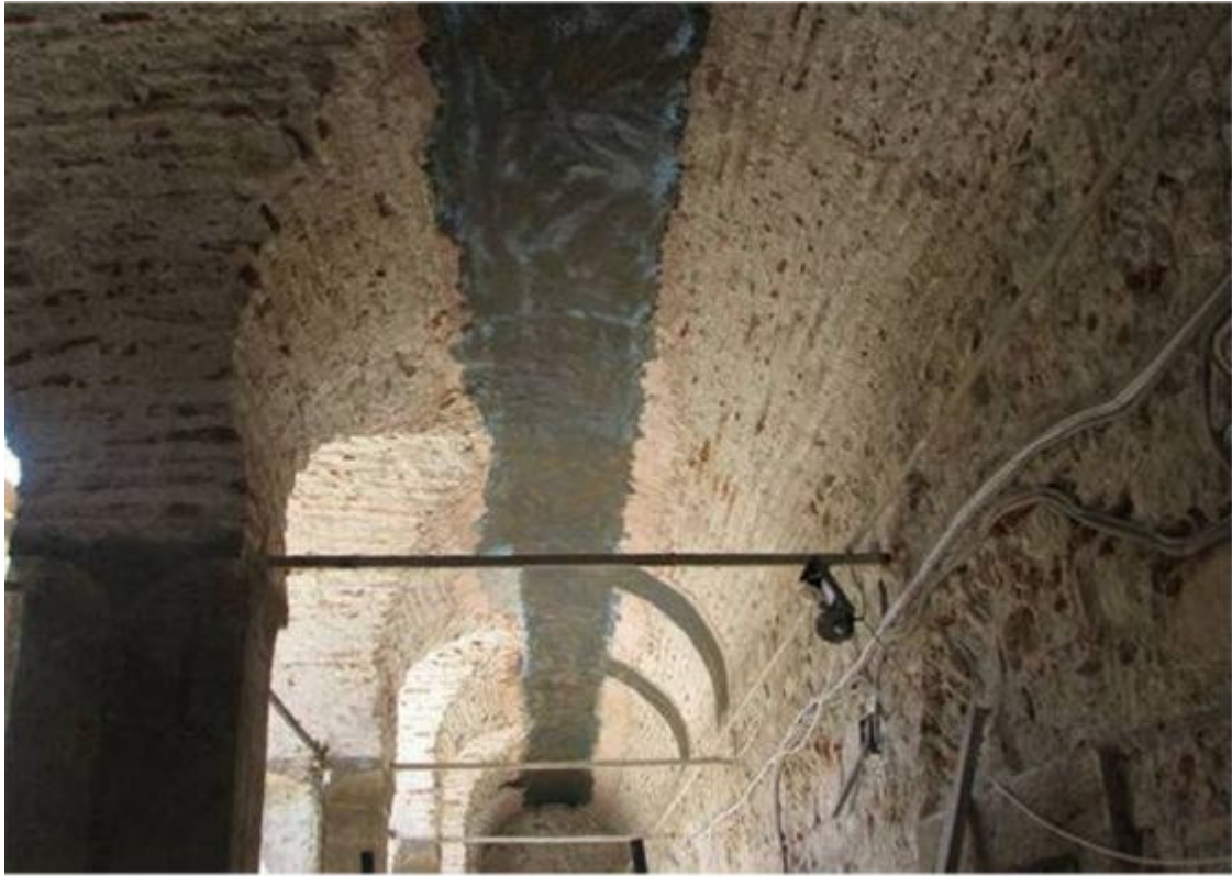
Figure 11. FRP applications under the vaults.
