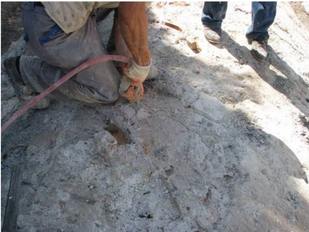
Figure 14. Application of injection materials above the vaults.
