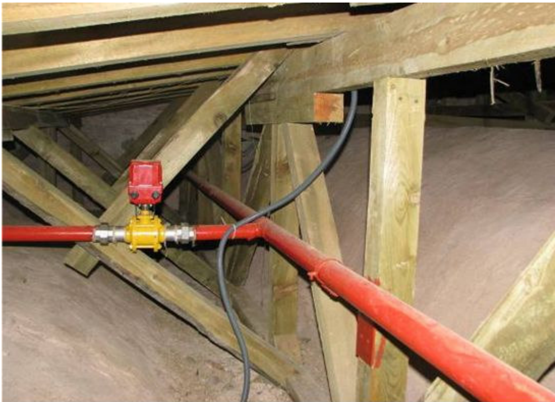
Figure 18. Automatic gas extinguishing system (FM200) under the wooden roof.
