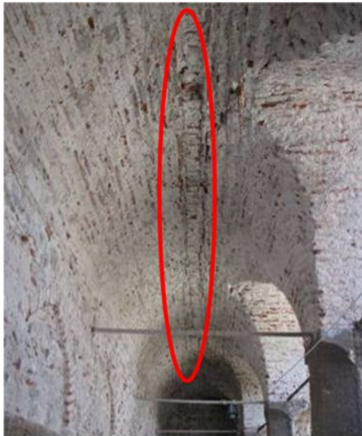
Figure 7. In-situ cracks under vaults in North-South direction.
