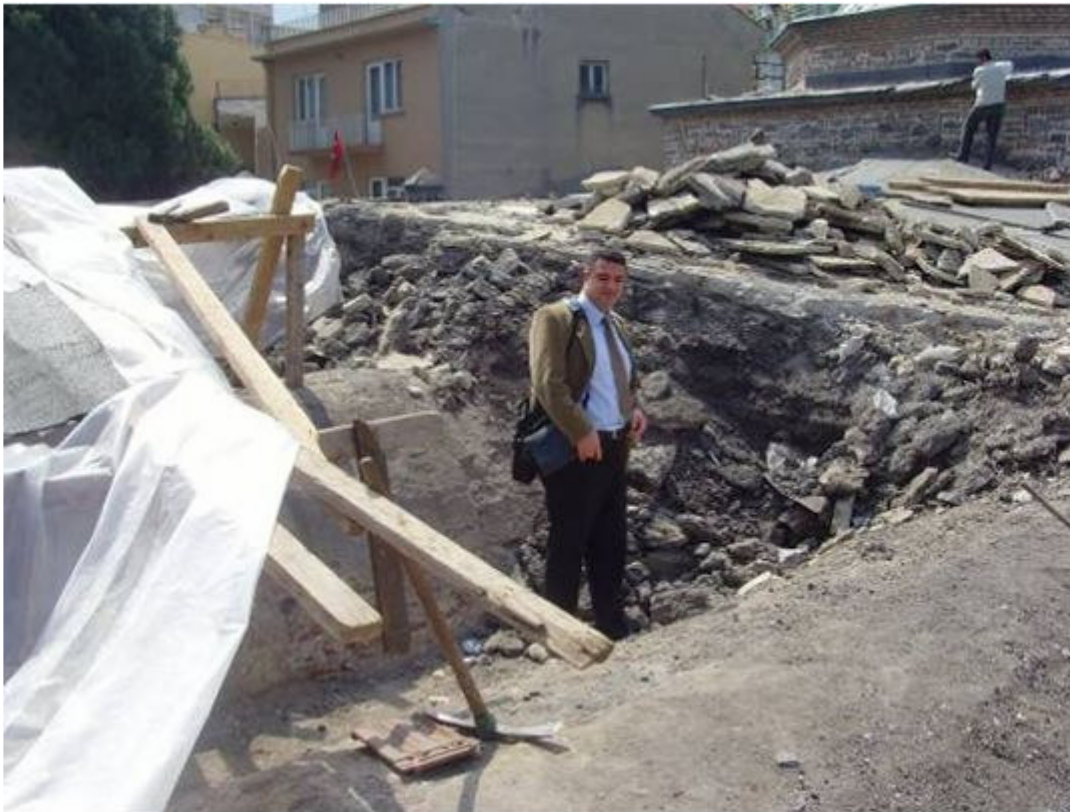
Figure 4. Different materials filling between and above the vaults.
