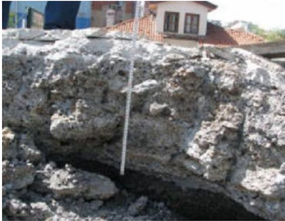
Figure 5. Layers of filling materials on vaults.
