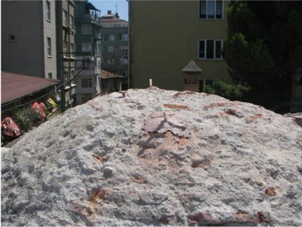
Figure 13. Application of injection materials above the domes.
