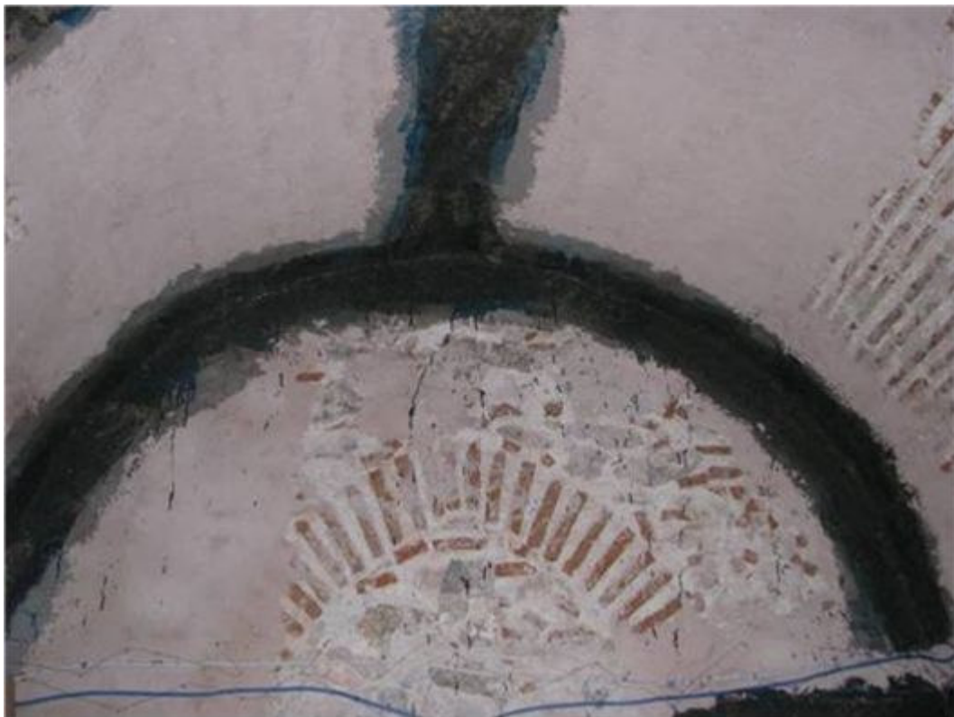
Figure 12. FRP applications at edge of the vaults.
