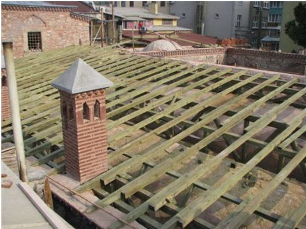
Figure 16. Perspective view of new wooden roof system.
