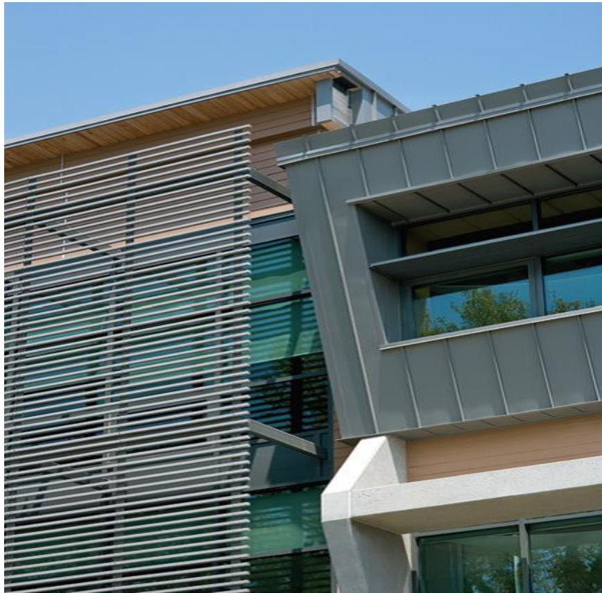
Fig. 10. Luis & Clark's office building, for the Missouri Ministry of Natural Resources, has been well integrated into solar control for glass envelope. (Source: BNIM)
