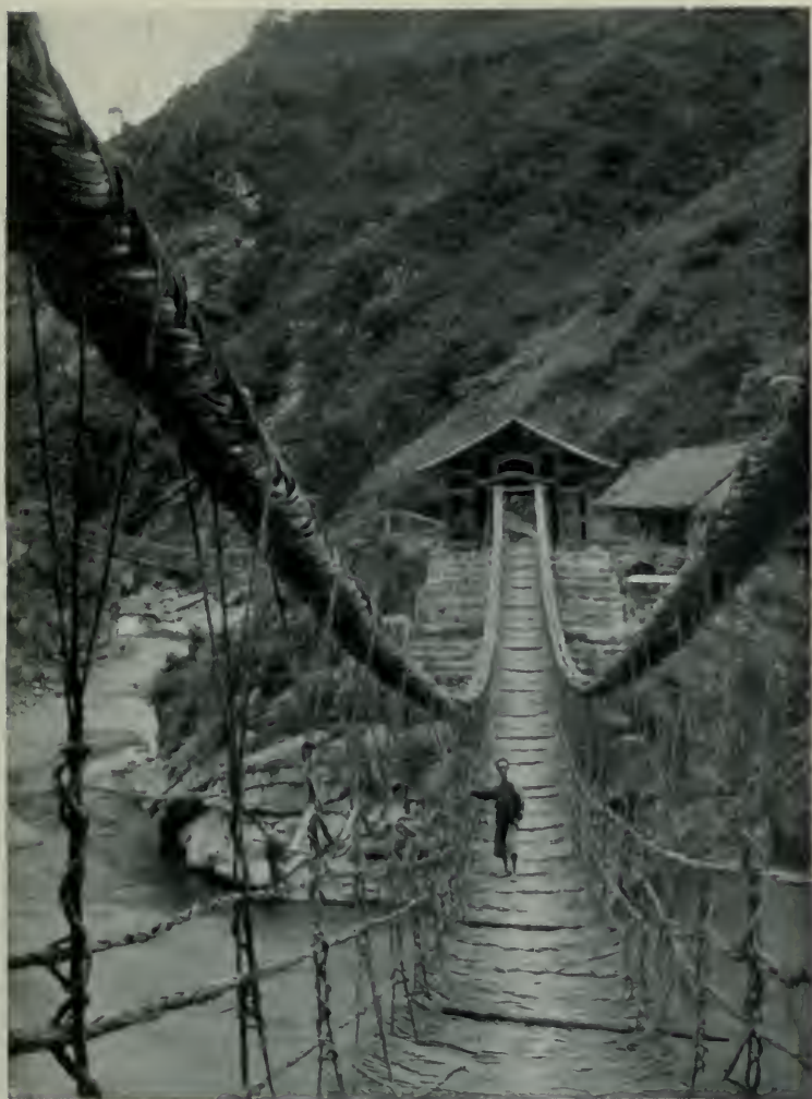
A BAMBOO SUSPENSION BRIDGE 70 YDS. LONG
