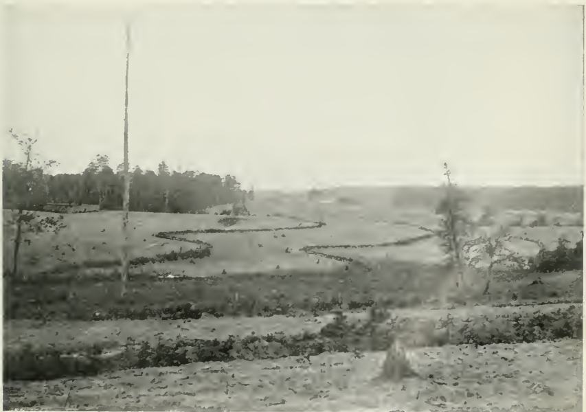
PLATE 4b. THESE TERRACES, ALTHOUGH WELL LOCATED, ARE TOO FAR APART, THE RISE BETWEEN THEM BEING TOO GREAT. AT LEAST ONE INTERVENING TERRACE SHOULD HAVE BEEN CONSTRUCTED.
