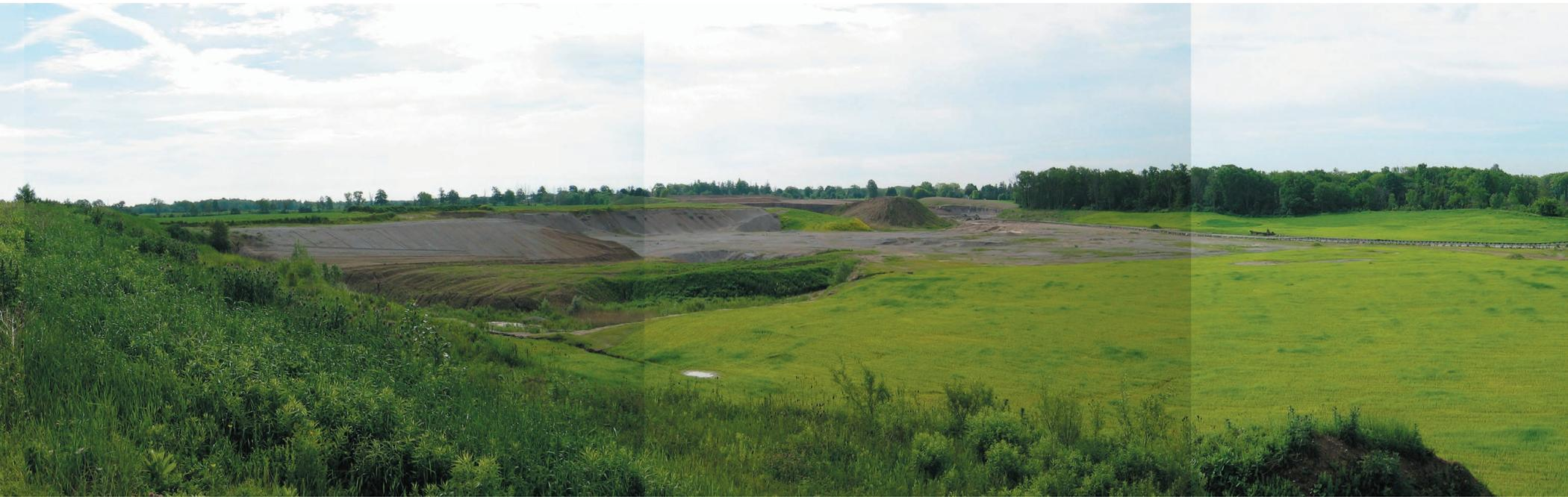
Fig. 123 | Looking south into southeastern extraction area. The Altrieve Lake and Forest (E.S.P.A. # 56) is the distance. Quick growing grasses are planted to prevent erosion as phases of extraction move to a different area of the site.
