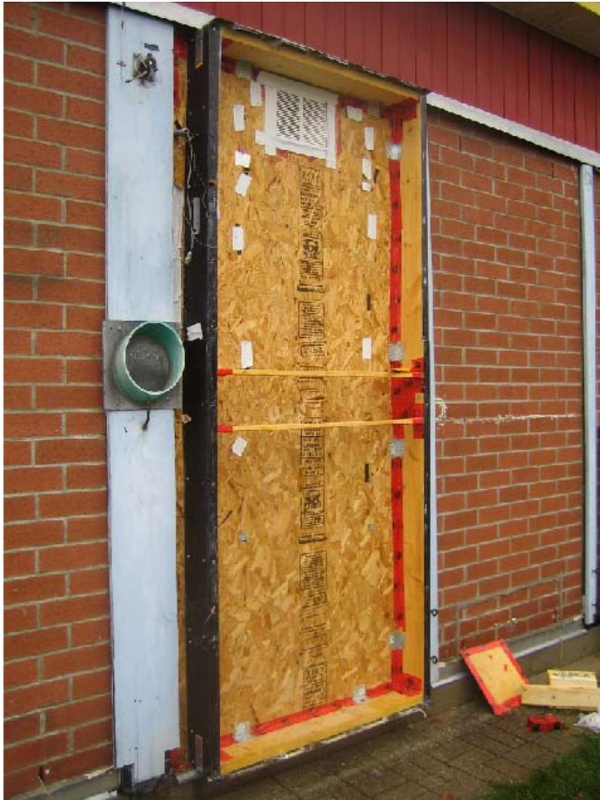
**Figure 4.6:** View of the BEG Hut east wall with the plenum box installed
