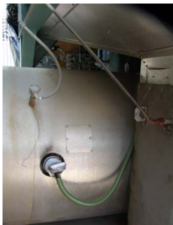
Figure 17a. Sample port with heated line to equipment. RTO is to the right. Equipment is behind large duct.
