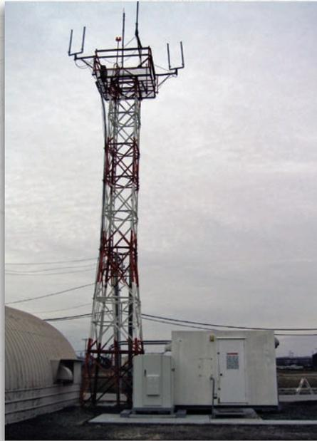
*A 1-kW fuel cell system has been providing power for this Federal Aviation Administration radio tower near Chicago for more than 3 years. The hydrogen storage and delivery system and fuel cell itself are all contained in the smaller cabinet closer to the tower.*
