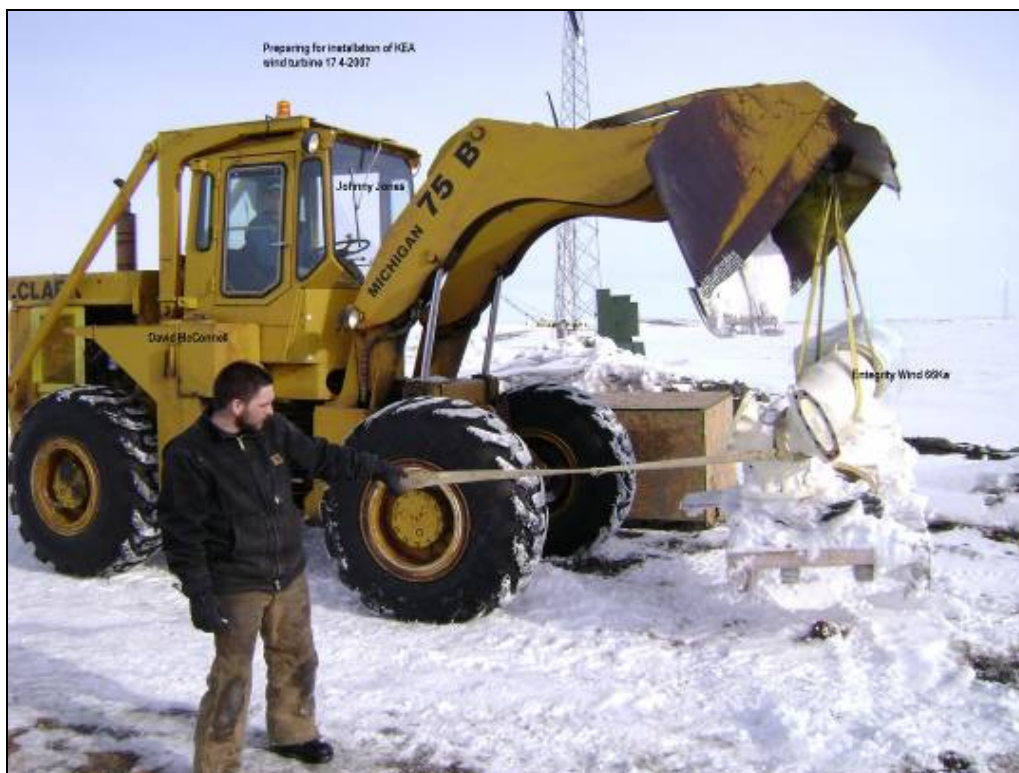
Figure 4. Preparing Turbine 17 Nacelle for Installation
