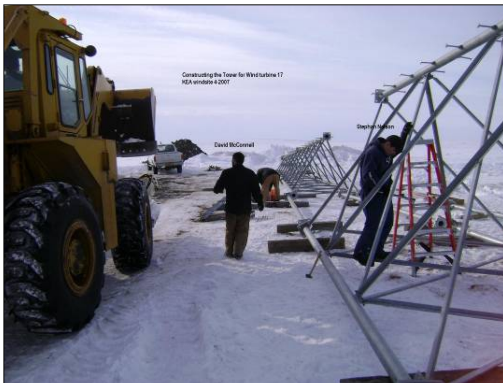
Figure 3. Assembling Turbine 17 Tower
