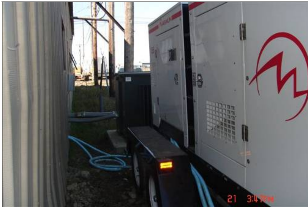
Figure 10. Backup Generator Set Up During SCADA Installation
