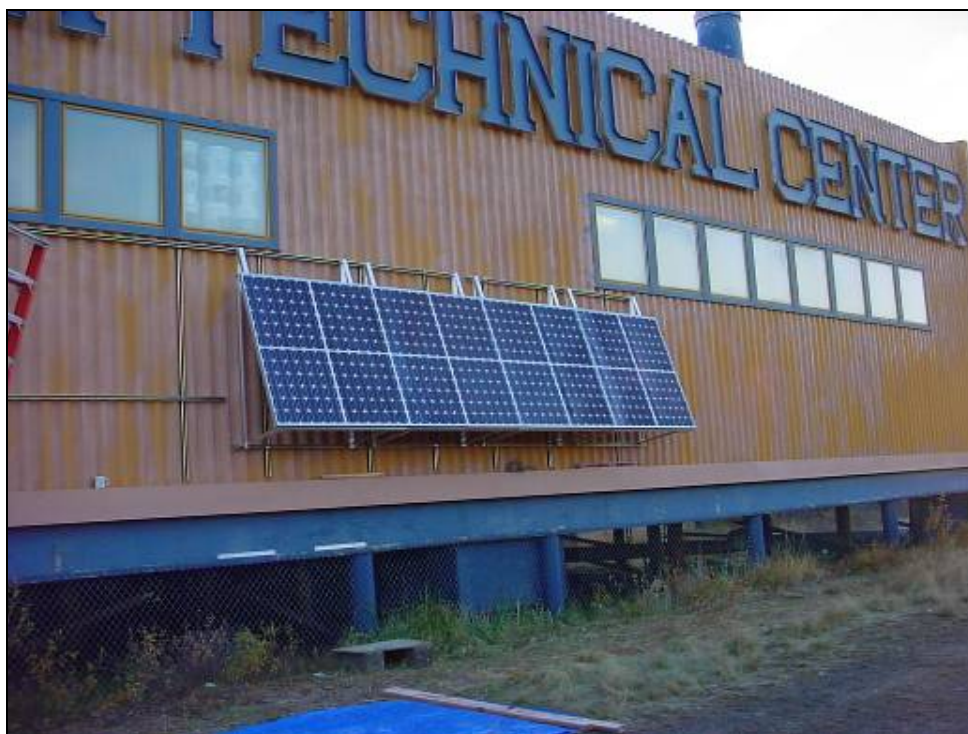
Figure 8. Completed Installation of Solar Panels at the Alaska Technical Center
