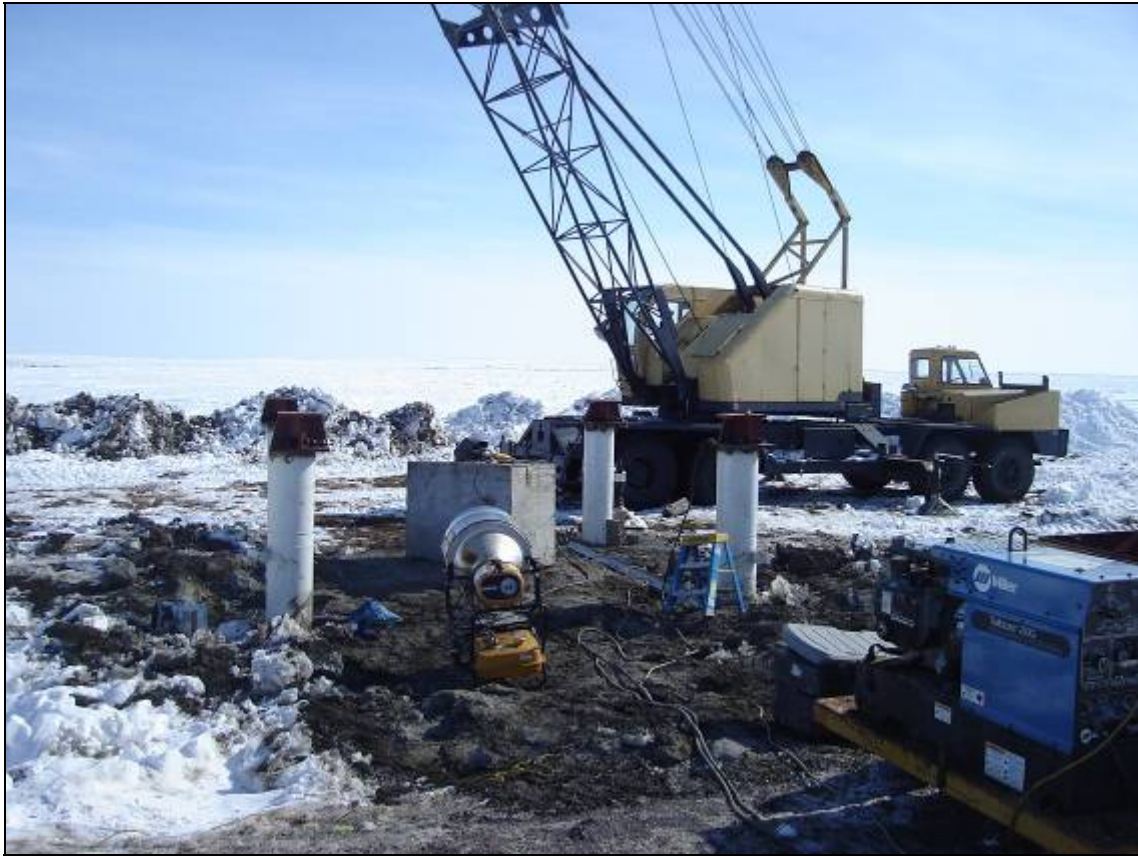
Figure 19. The V-15's Four-Legged Lattice Tower Piling Foundation
