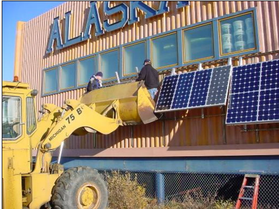
Figure 7. Installing Solar Panels at the Alaska Technical Center
