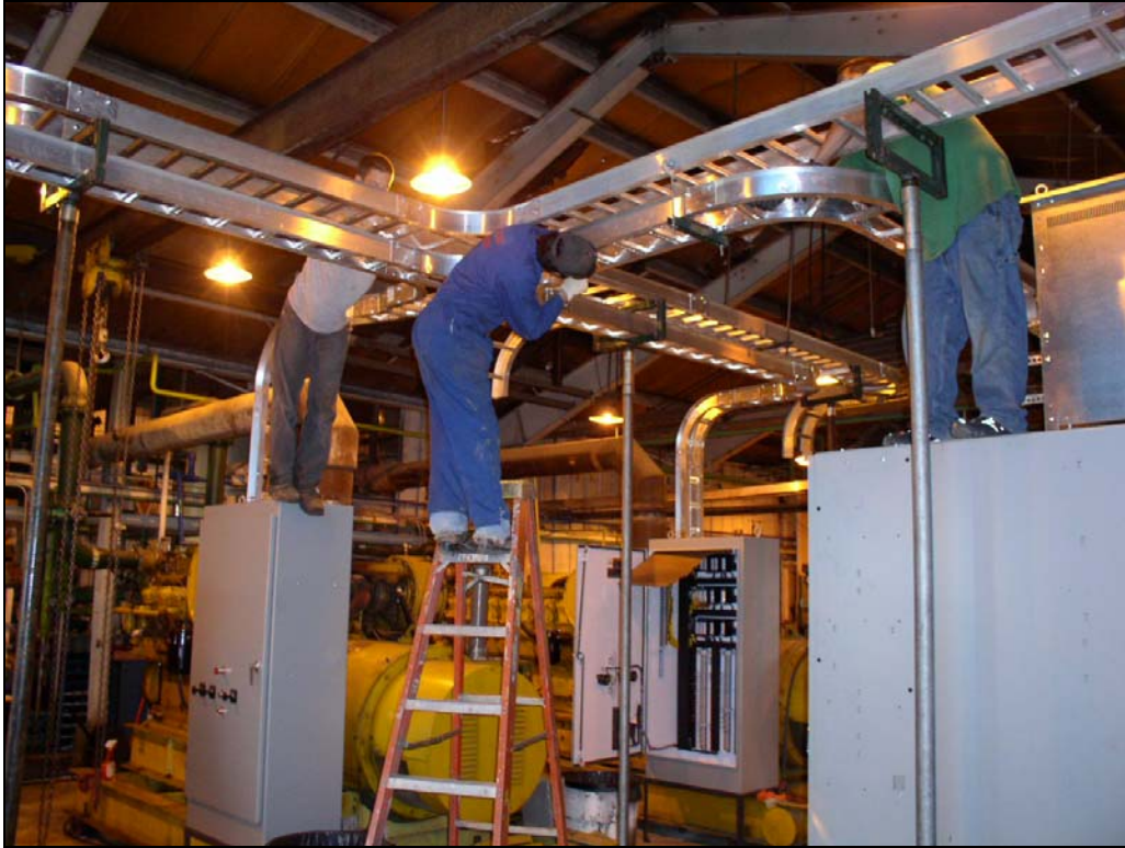
Figure 16. Installing Cable Trays in the Power Plant
