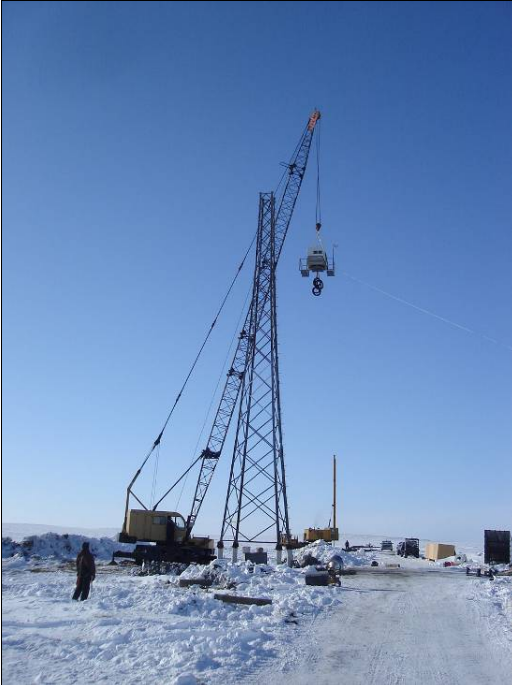
Figure 20. Mounting the V-15 Nacelle on the Tower
