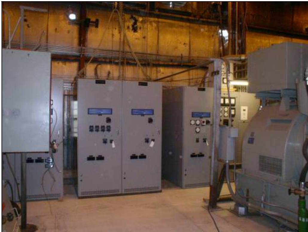
Figure 18. Installation of New Switchgear in Newer Section of Plant
