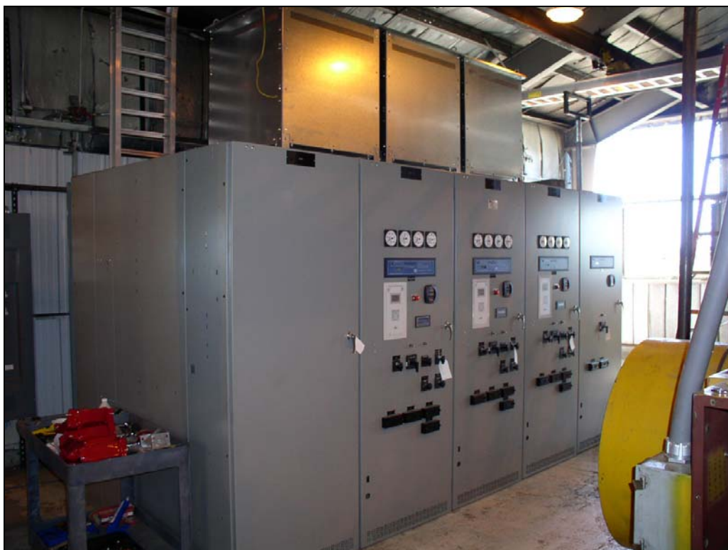
Figure 15. New Switchgear in Place and Leveled
