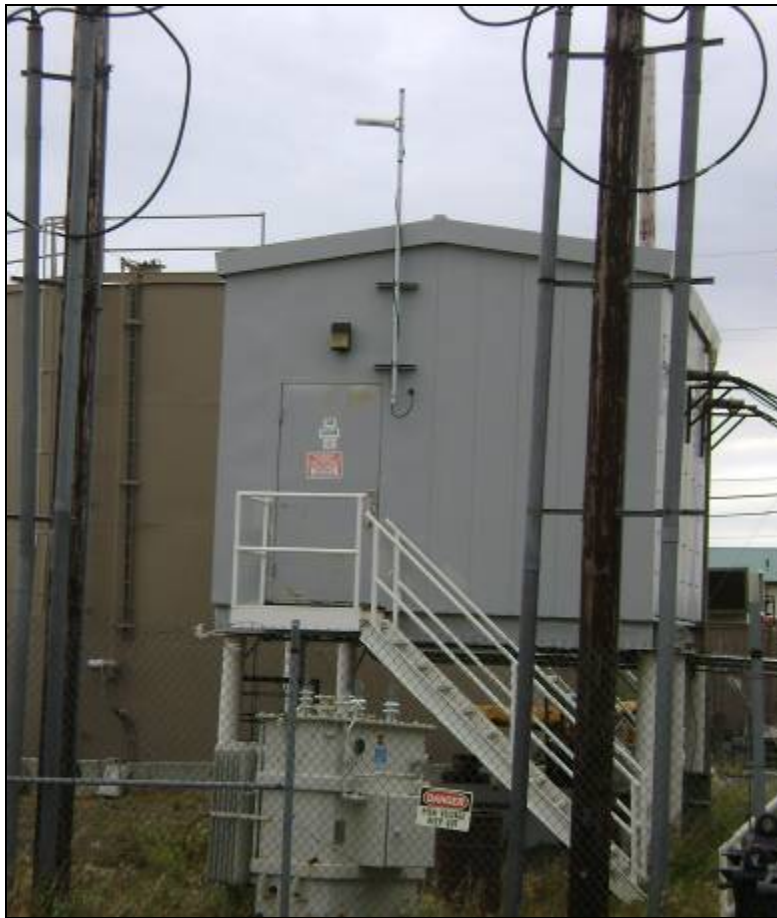
Figure 17. Antenna for High-Speed Radio Link Mounted on Substation Building
