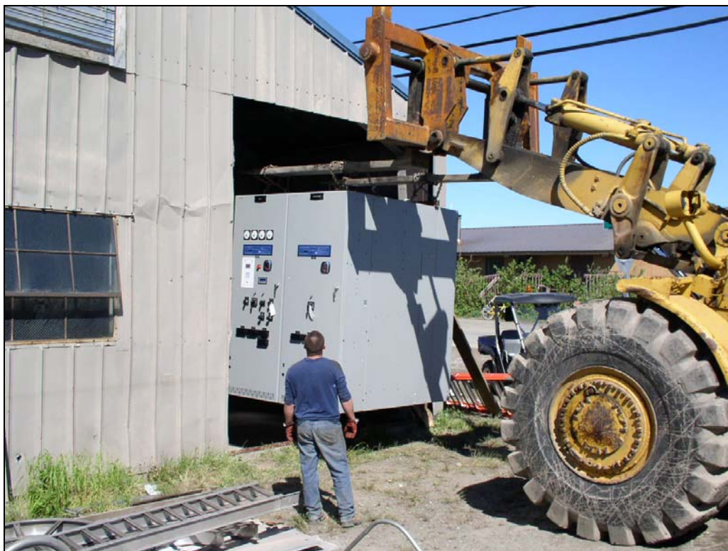
Figure 14. Installing New Switchgear in Old Section of Power Plant
