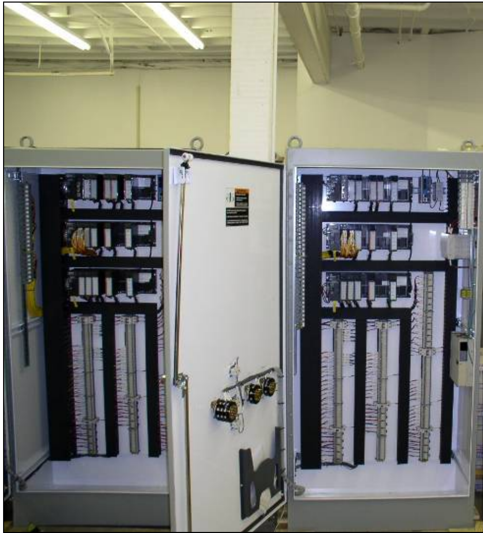
Figure 9. Diesel Engine PLC Panels from EPS
