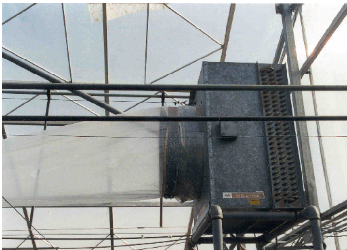
Photo 4. Modine heater with poly tube.
