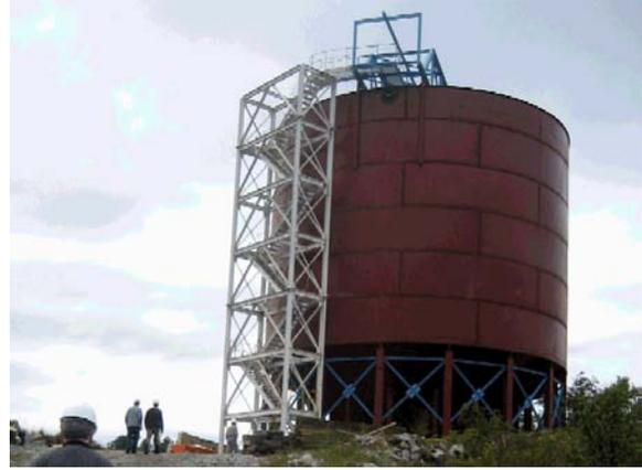
Figure 44. Paste thickener used to further thicken wastes for disposal.
