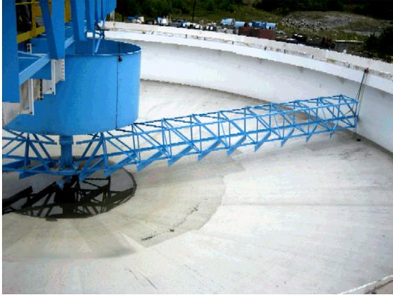
Figure 43. Static thickener used to thicken solids and clarify process water.
