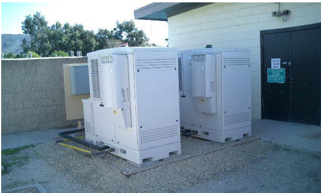
Fuel Cell Unit Numbers 315 and 317, Installed at Swimming Pool, Pt. Mugu.
