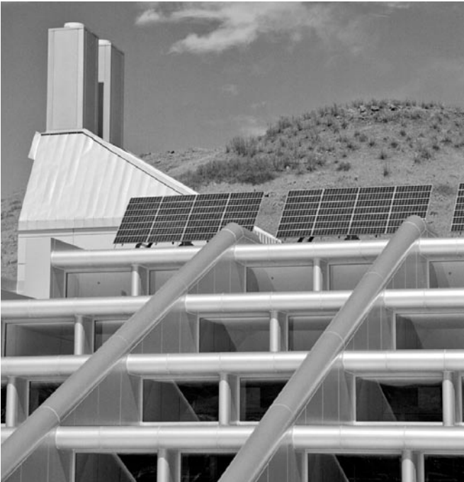
This energy-efficient laboratory building, built in Colorado in the 1990s, faces south and makes use of daylighting, evaporative cooling, and advanced heat recovery systems; the photovoltaic modules on the roof feed electricity into the local grid.
