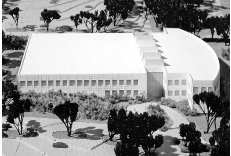
An artist's rendition of the EPA National Computer Center in Research Triangle Park, North Carolina; the building will include a 100-kW roof-integrated PV system for electricity generation.
