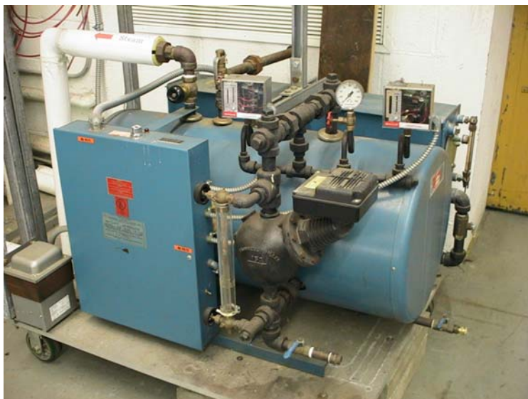
Figure 4. Electric Steam Generator
