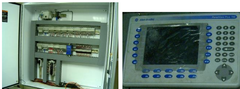
Figure 46. System Control Panel and HMI Display Installed at REP
