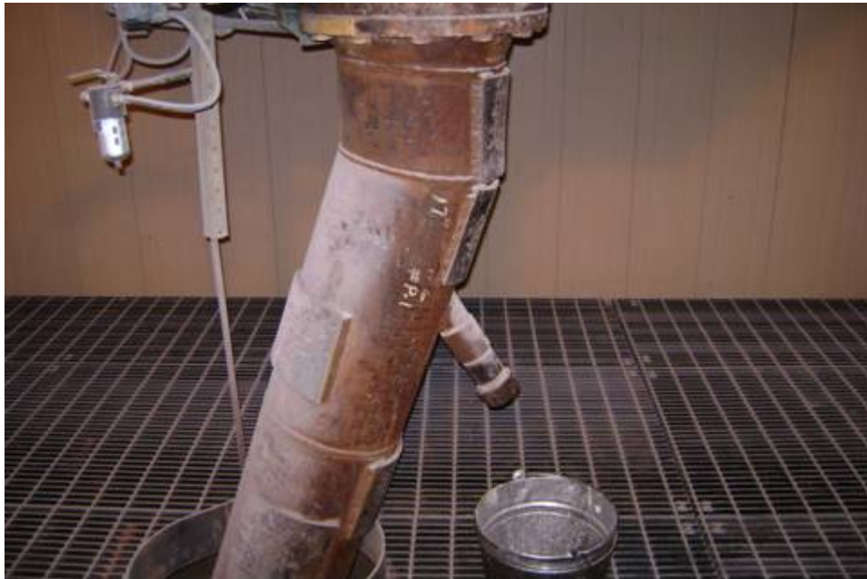
Figure 18: Sampling of Economizer Ash from a Downcomer
