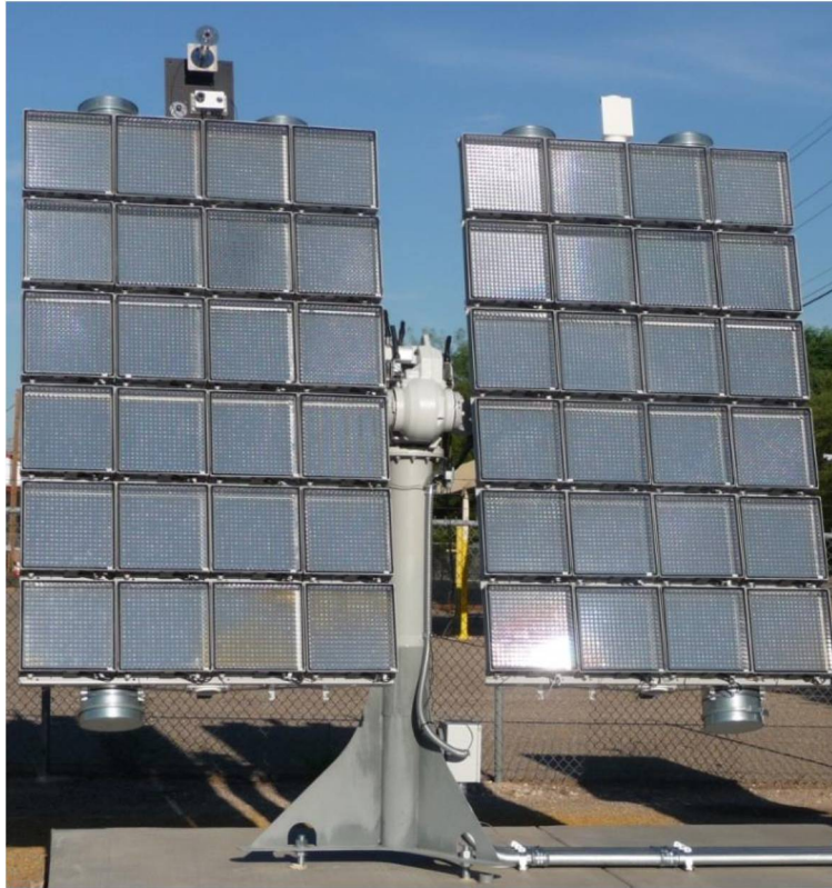
Figure 1. Semprius first 1kW HCPV RD&D system installed at Tucson Electric Power in AZ.
