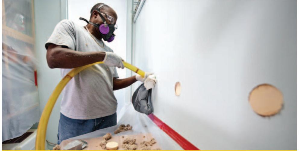
A weatherization worker adds insulation to walls in rooms that have been masked off from the rest of the unit. Healthy homes experts are contributing to the *Standard Work Specifications for Multifamily Energy Upgrades* to address occupant and worker safety issues. Photo by Dennis Schroeder, NREL/PIX 17964
