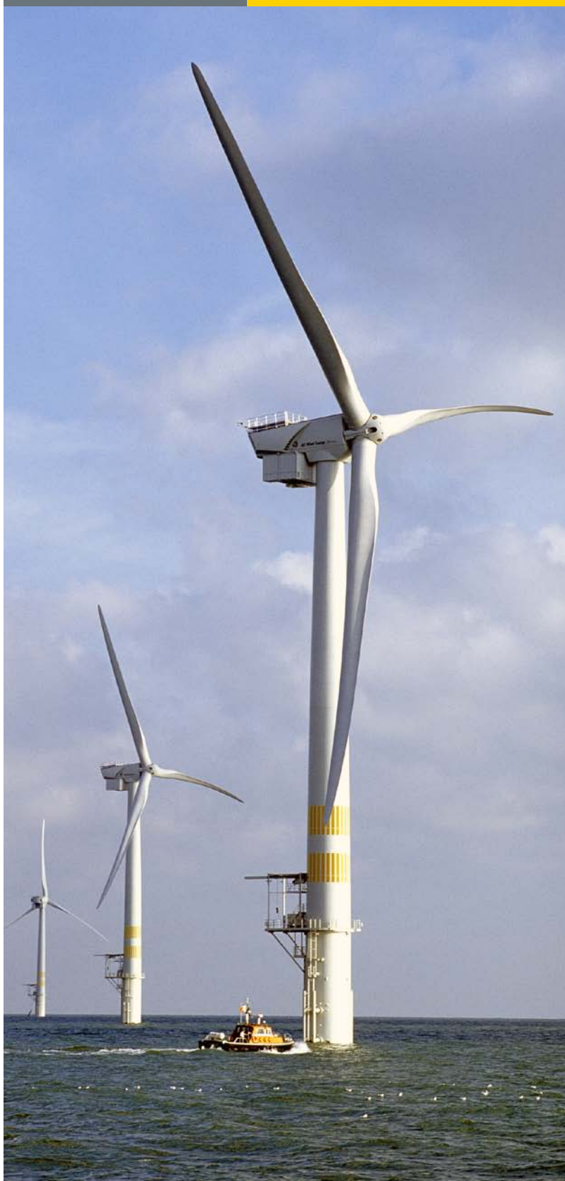
3.6-MW GE Wind turbine at Arklow Bank offshore wind facility near Arklow, Ireland. Photo from GE Wind Energy All Rights Reserved ©2003, NREL/PIX 13160
