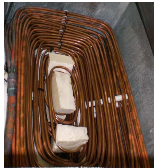
Figure 3: Example of condenser coil configuration to allow for adequate drainage of liquid refrigerant
