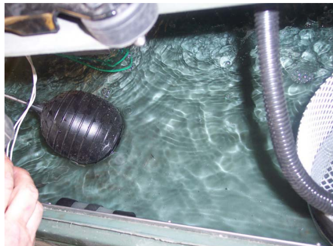
Figure 8: Float to adjust water sump level
