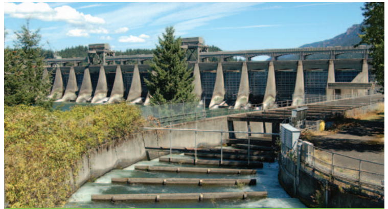
The Bonneville Dam on the Columbia River between Washington and Oregon provides safe passage to migratory fish via its fish ladders while maintaining a capacity rating of more than 1,000 megawatts. Photo from iStock/4200712
