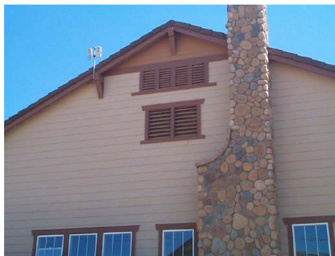
Figure 11: For this house the upper set of louvers is for the outside air intake; the lower pair is for attic ventilation.
