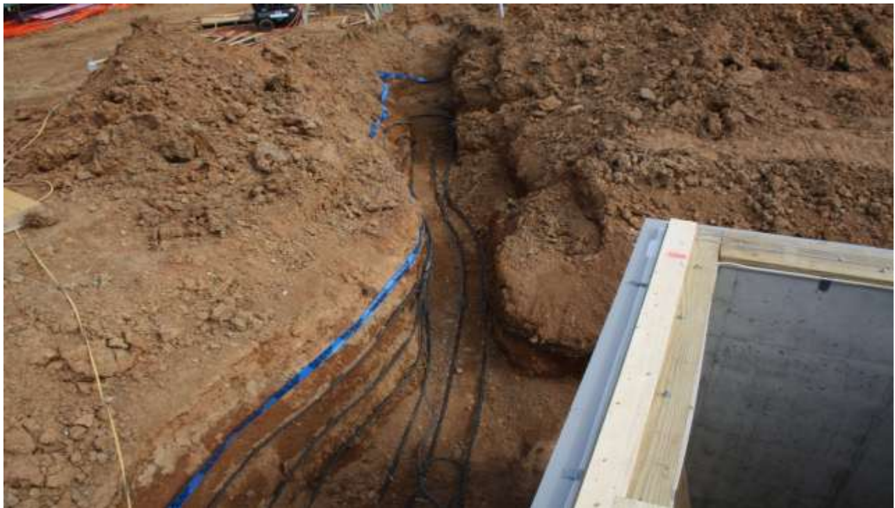
Figure 2.9. HGHX installed in a utility trench.
