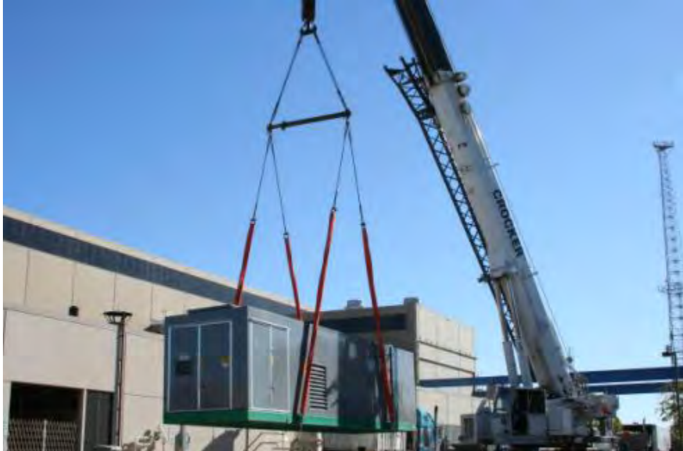
Hydrogen station being lifted by crane from delivery truck at the University of Texas Pickle Research Center, November 2008
