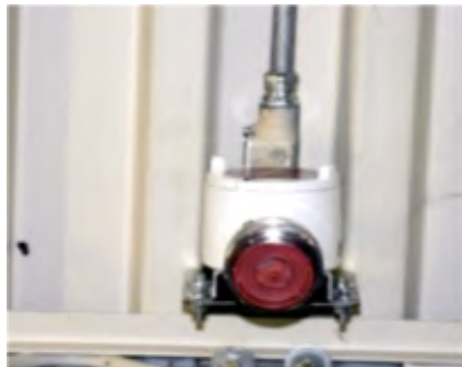
Hydrogen Gas Sensor (mounted at highest point in the ceiling)
