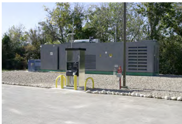
Hydrogen fueling station. University of Texas Pickle Research Center, Austin, TX. Reformer, processing, storage, etc., etc.. Can produce 60 kg per day. 2009.
